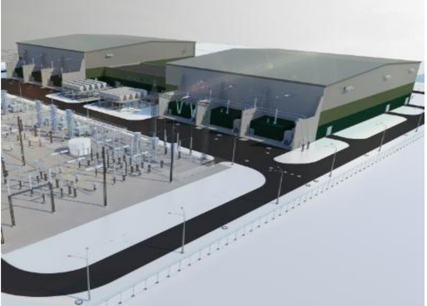
Image D.7 VSC converter station
