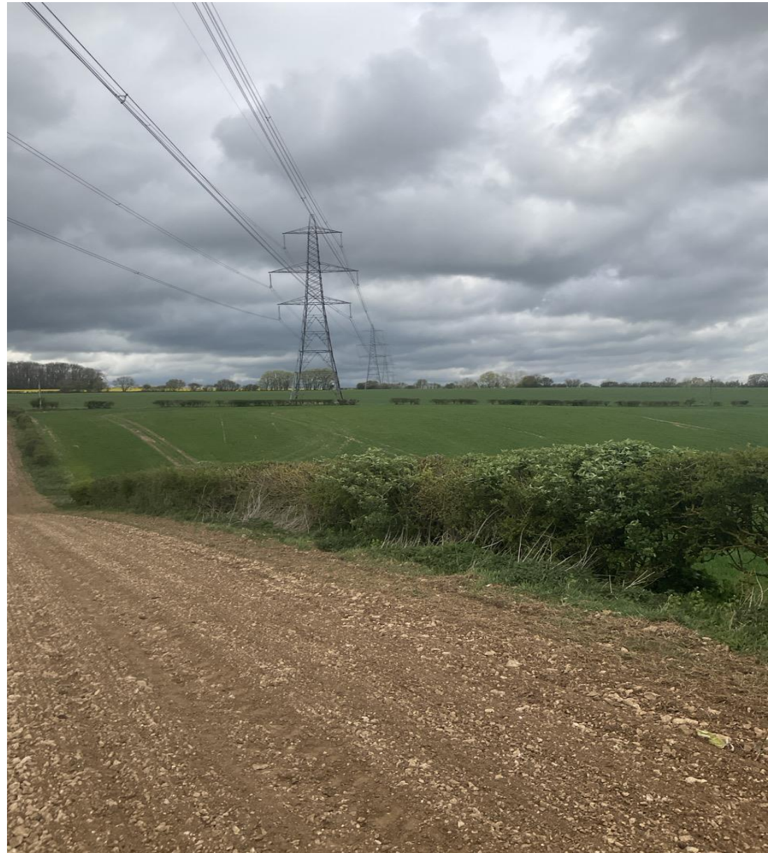
GGP-GI-Pt-36 Infrastructure General view of overhead line infrastructure bisecting fields 36a
