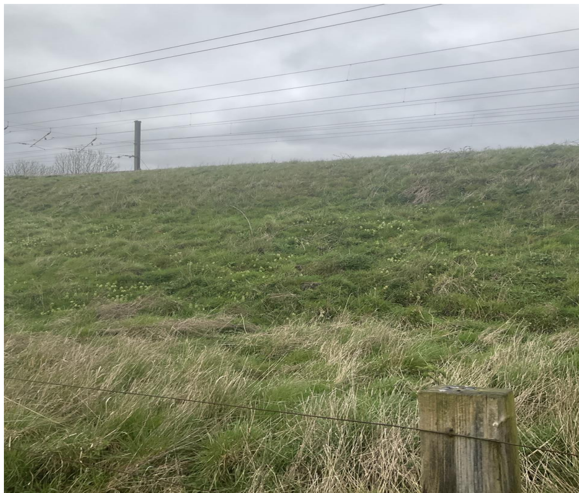
GGP-GI-Pt-55 Infrastructure / Slope General view of railway embankment 55a
