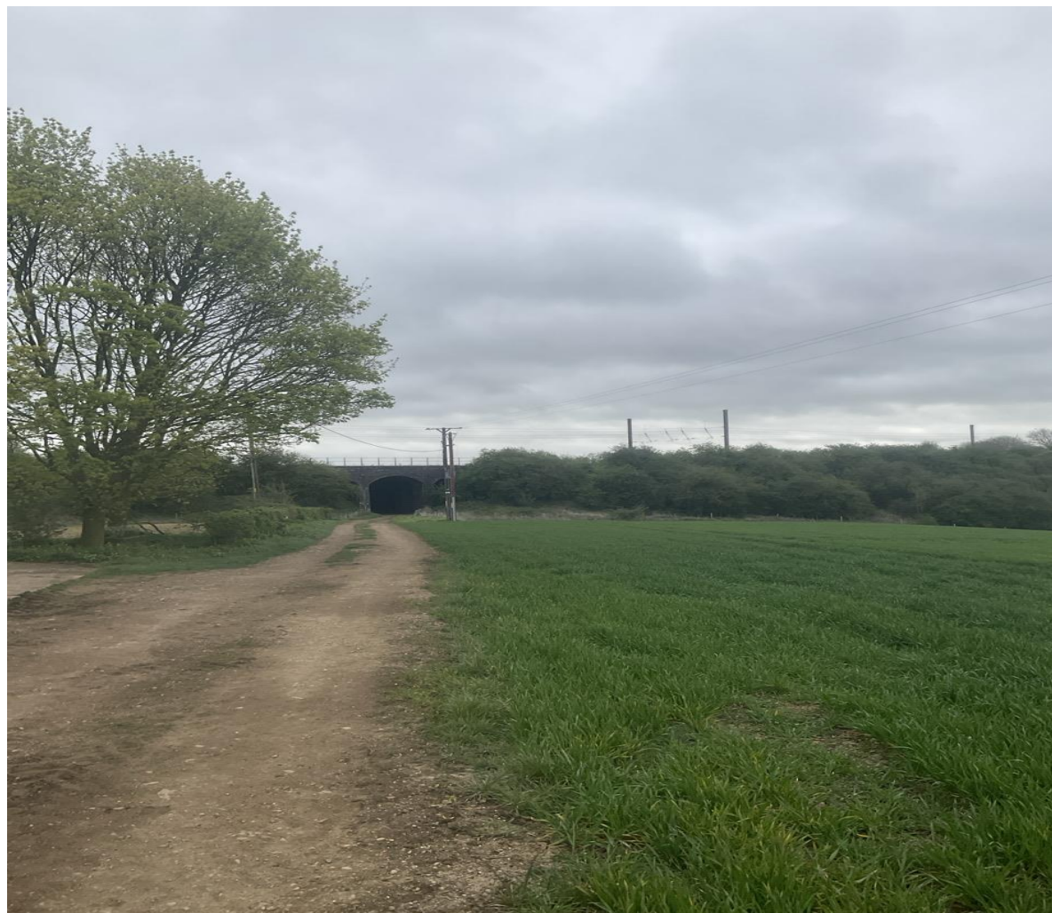
GGP-GI-Pt-56 Utility General view of existing overhead infrastructure 56b
