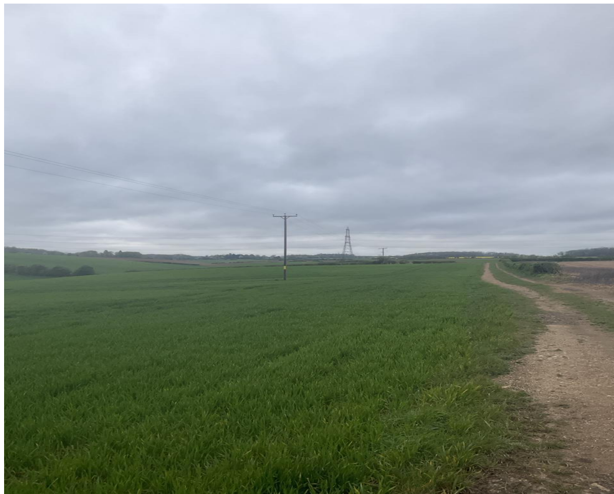
GGP-GI-Pt-56 Utility General view of existing overhead infrastructure 56a
