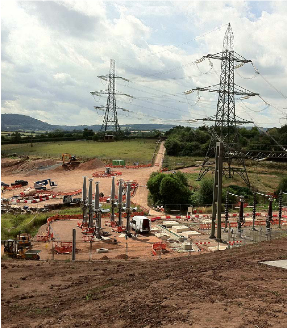
The undergrounding of electricity cables at Ross-on-Wye
