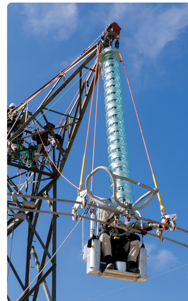
An overhead line operative working at height
