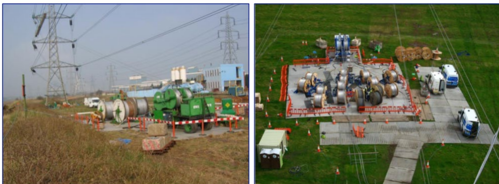
Figure 2 - Machinery associated with conductor pulling at stringing areas
