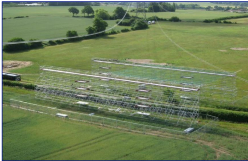
Figure 3 - Example of scaffold crossing protection
