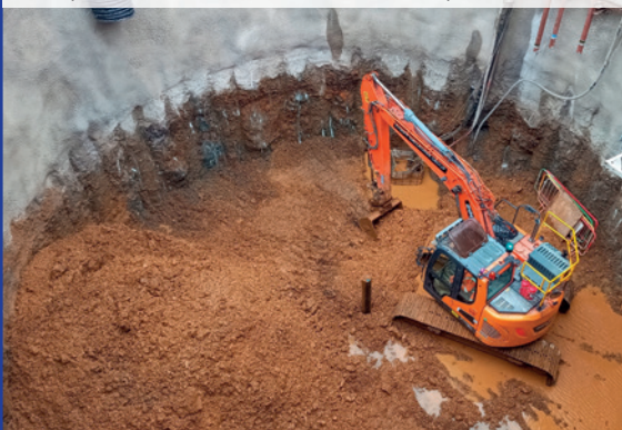
Reception shaft at 15m excavation depth
