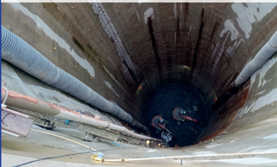
Reception shaft at 49m excavation depth
