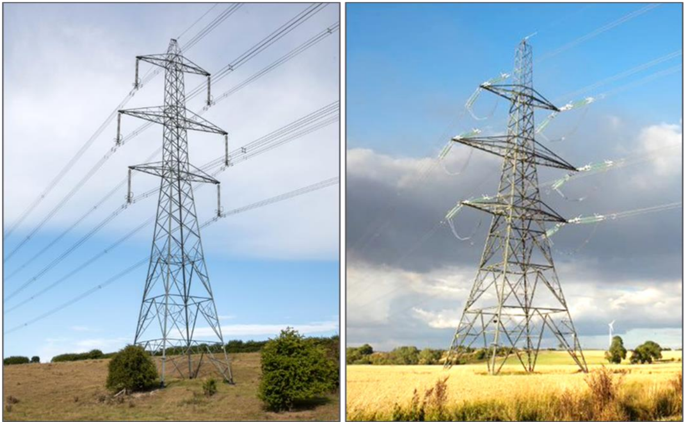
Image 4.2 Typical suspension pylon (left) and typical tension pylon (right)
