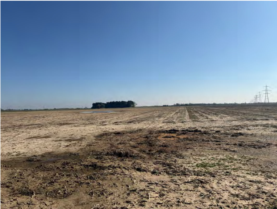
Photograph 8: Looking south east from Marsh Road, along the existing overhead line.
