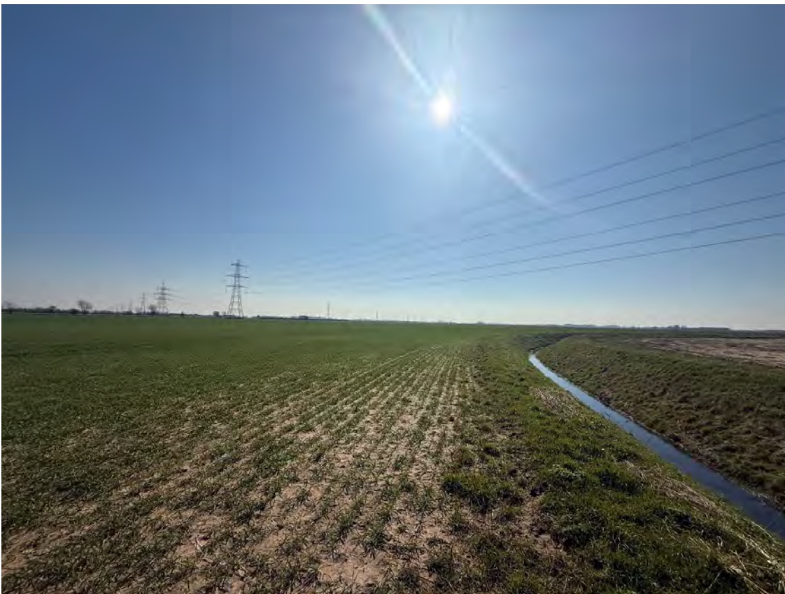
Photograph 15: Looking south west from the public footpath towards the existing overhead line and new substation location.
