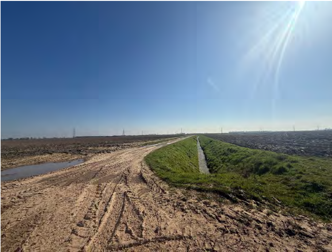
Photograph 2: Looking south east from Marsh Road across the New Weston Marsh Substation A location.
