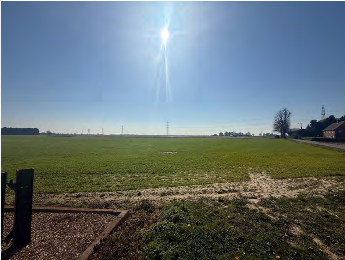
Photograph 10: Looking south from Marsh Road towards the existing overhead line and New Weston Marsh Substation A location.
