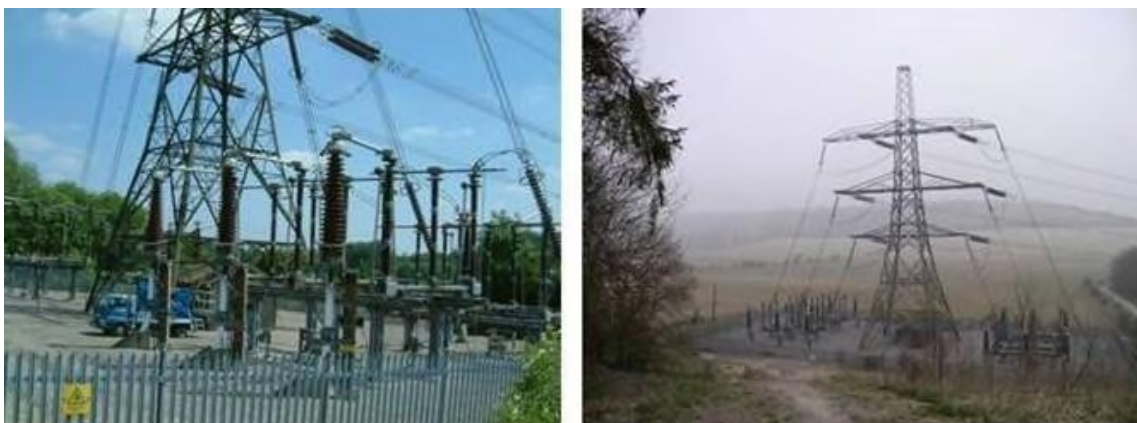
Figure C.5 – Cable Sealing End Compounds
