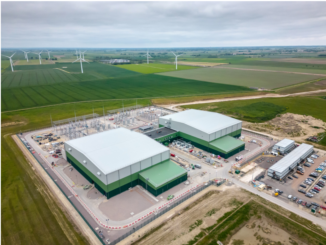
Figure 2.3.4: Converter Station Facility developed for the Viking Link Interconnector Project, illustrating a typical layout and scale of infrastructure
