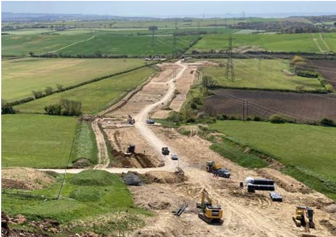
Figure 2.3.3: Typical Underground HVAC cable construction
