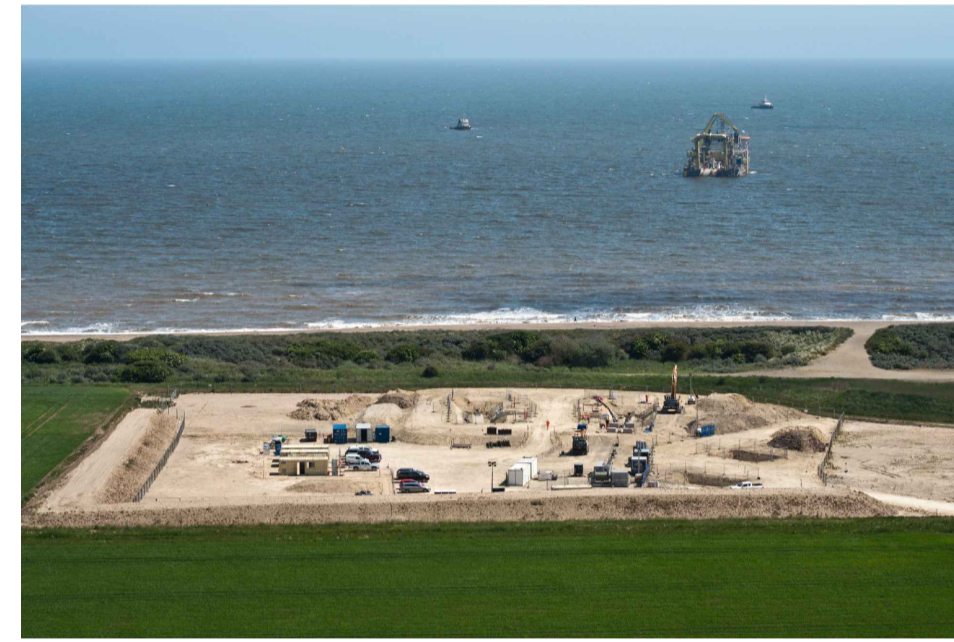
Example of a Trenchless Method Landfall Site (Triton Knoll, 2024)
