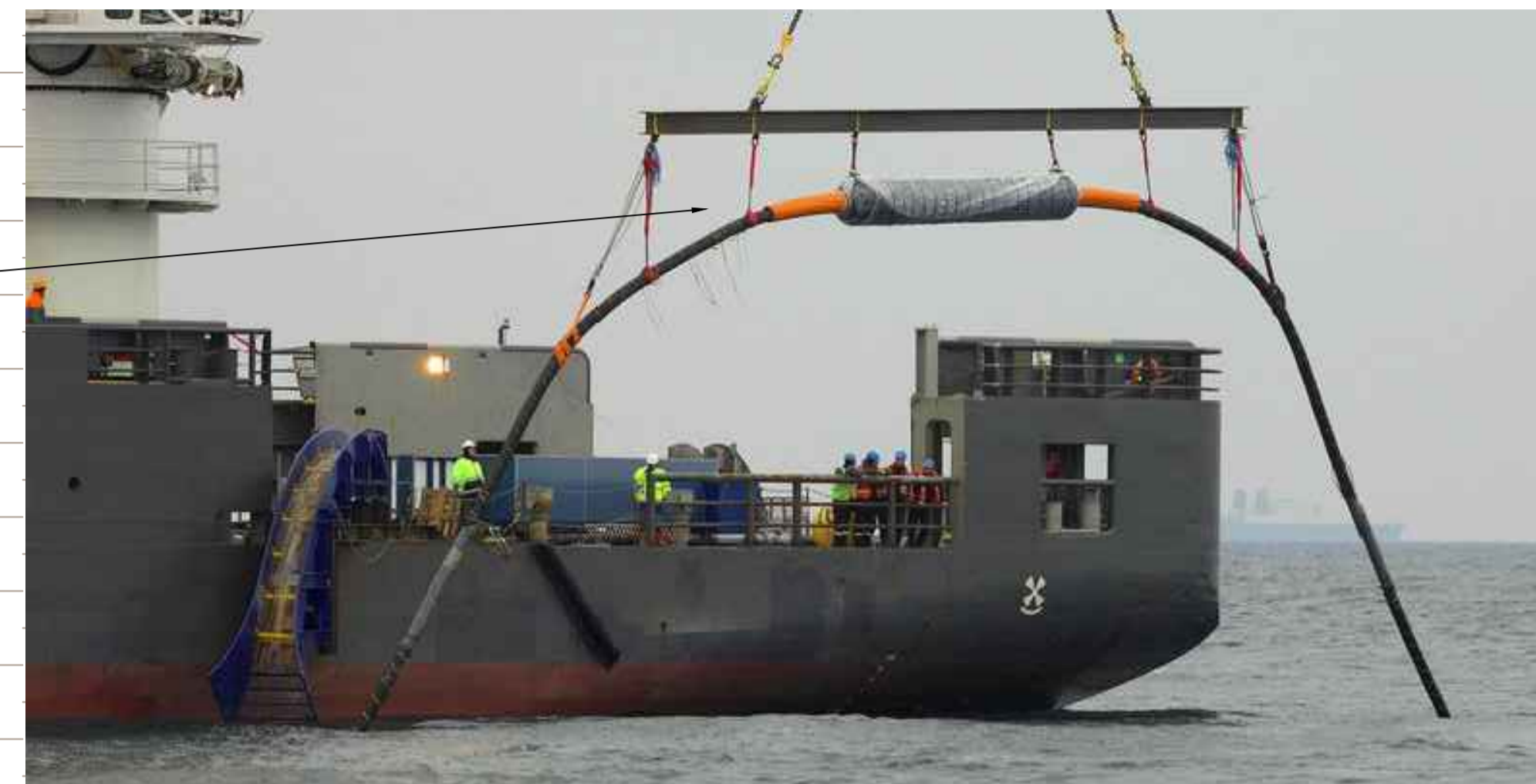
Cable joint lifted above the sea surface (NKT, date not known)
