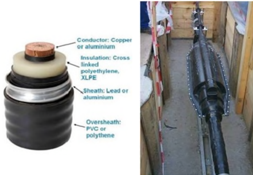
Figure C.4 – Cable cross-section and joint
