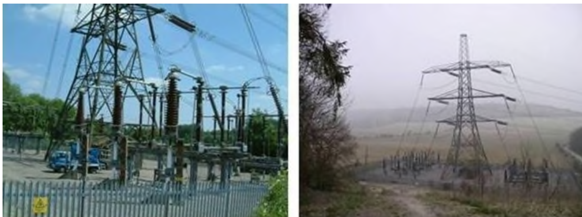
Figure C.5 – Cable Sealing End Compounds
