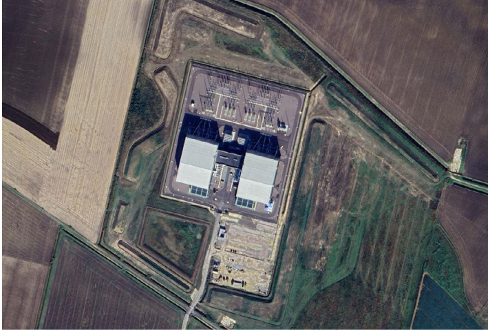
Figure 4.17 Viking Link converter station, Bicker Fen, Lincolnshire.
