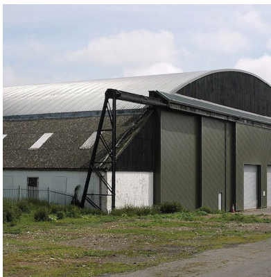
Figure 4.35 Curved roof design seen in an airfield building in Lincolnshire
