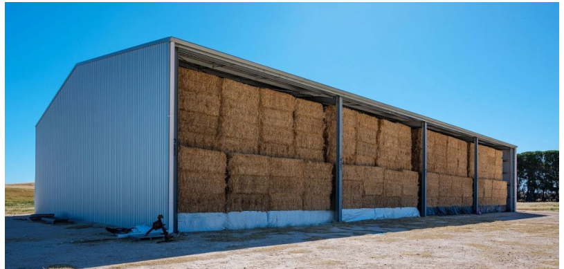
Figure 4.52 Hay bales stored under shed
