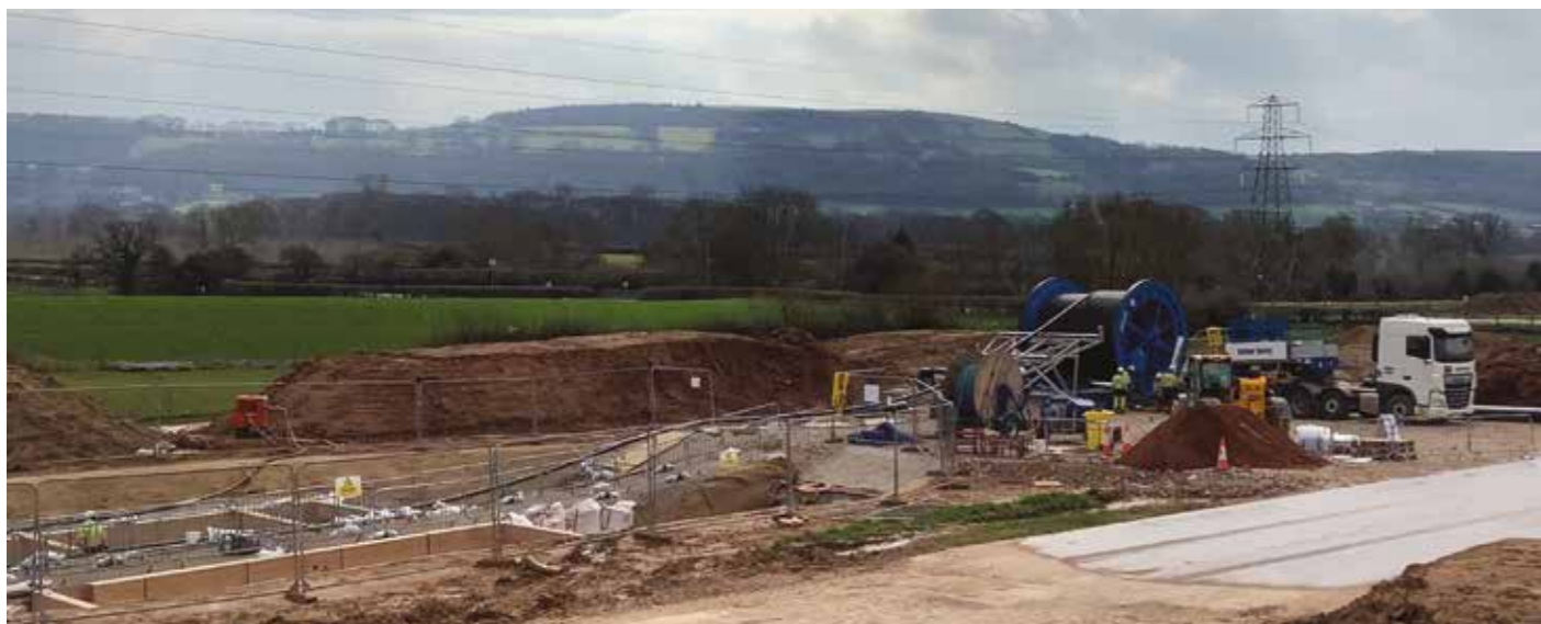
Figure 17 – The ducted method of cable laying
