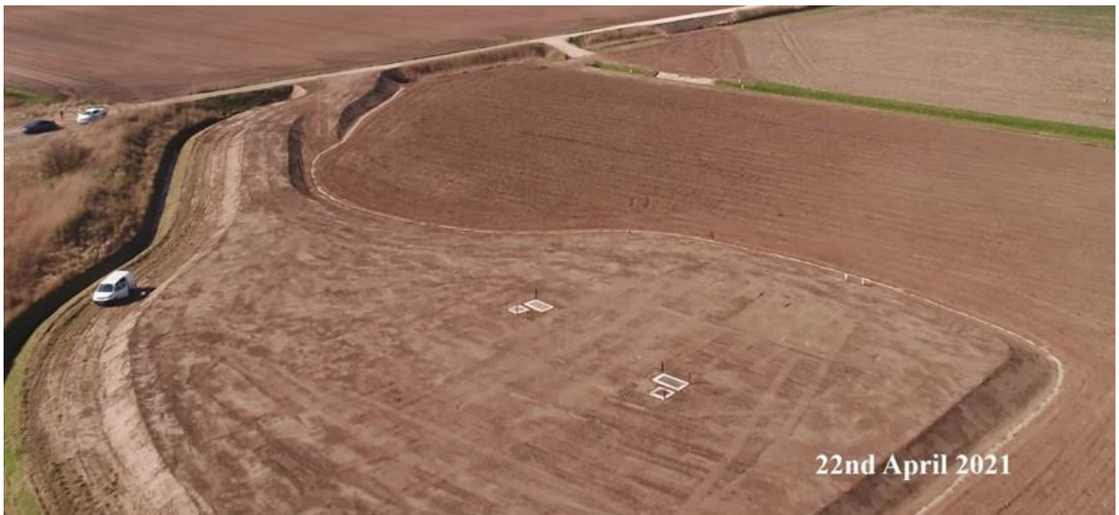
Plate 4-7 Illustration of a TJB raised platform
