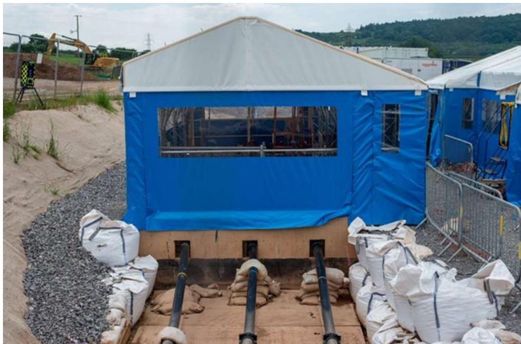
Plate 4-5 Cable joint bay
