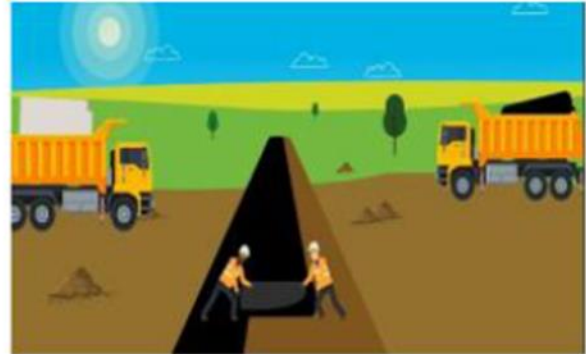
Step 2 A layer of synthetic material is installed to aid the removal of stone, where required, and to stabilise the stone layer for the haul route surface
