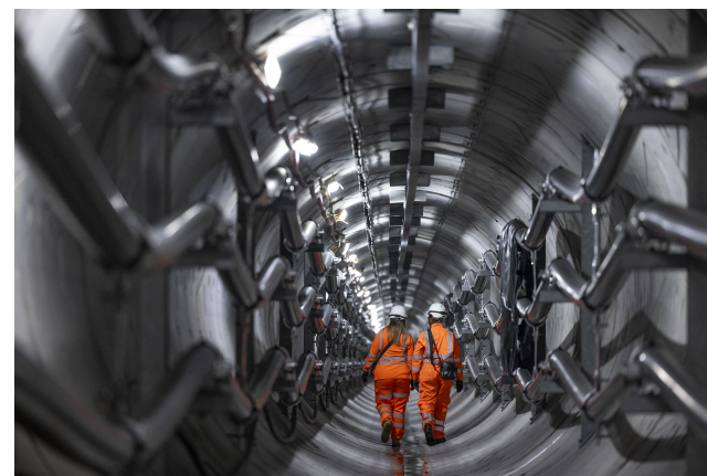
London Power Tunnels, UK
