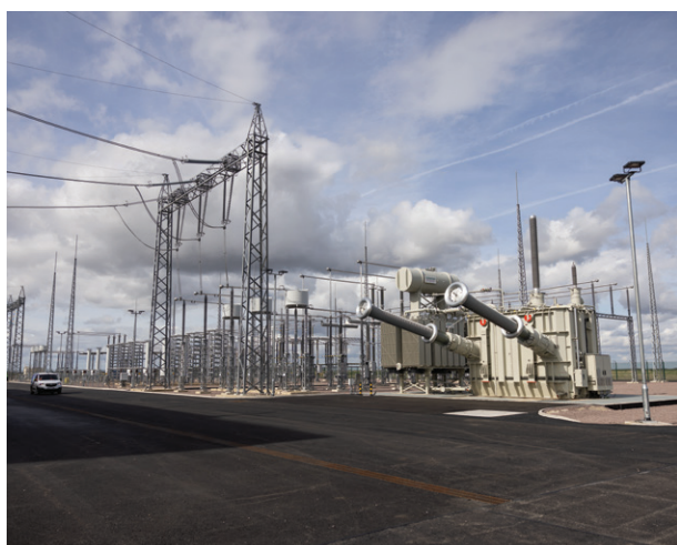
Example AC switching yard as part of converter station compound, pictured on Viking Link
