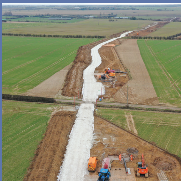
Example of haul road construction
