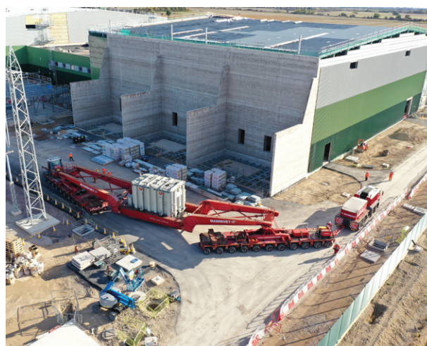
Delivery of transformer unit to the Viking Link project
