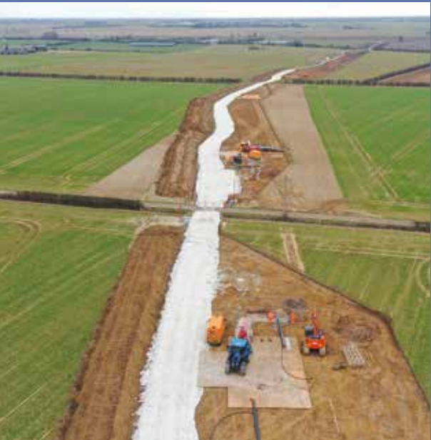
Example of haul road construction
