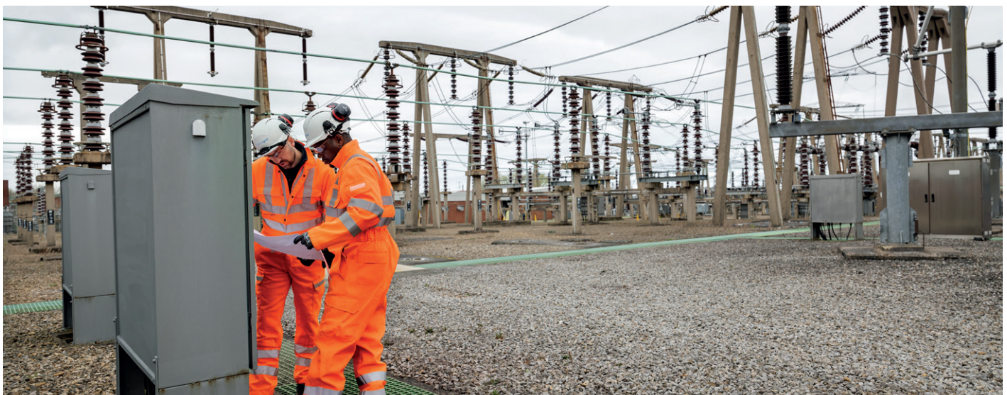
National Grid staff at work in a substation
