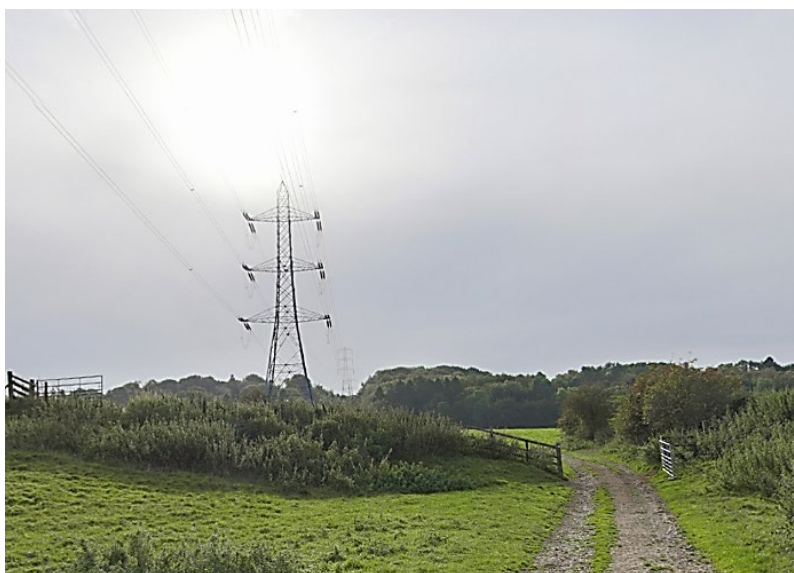
Figure 3: Visual intrusion presented by the ZF.2 overhead line and pylons
