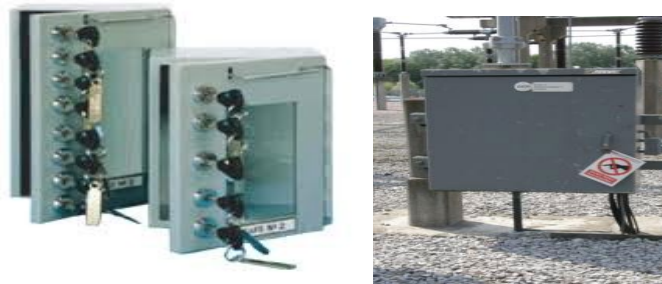
Figure 4.4A – Example of a Key Safe and safety precautions applied
