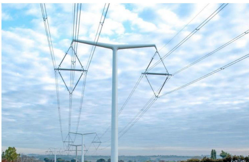
Image 5.9 Typical suspension T-pylon
