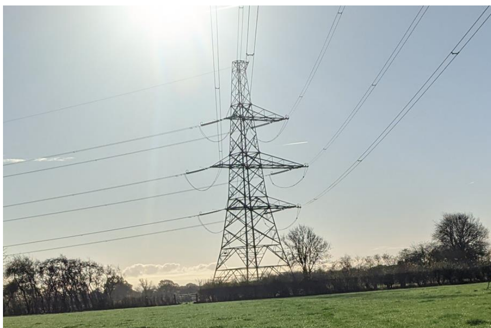
Image 5.12 Typical tension/angle lattice pylon 2
