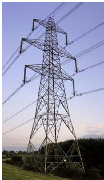
Image 5.10 Typical suspension steel lattice pylon 1
