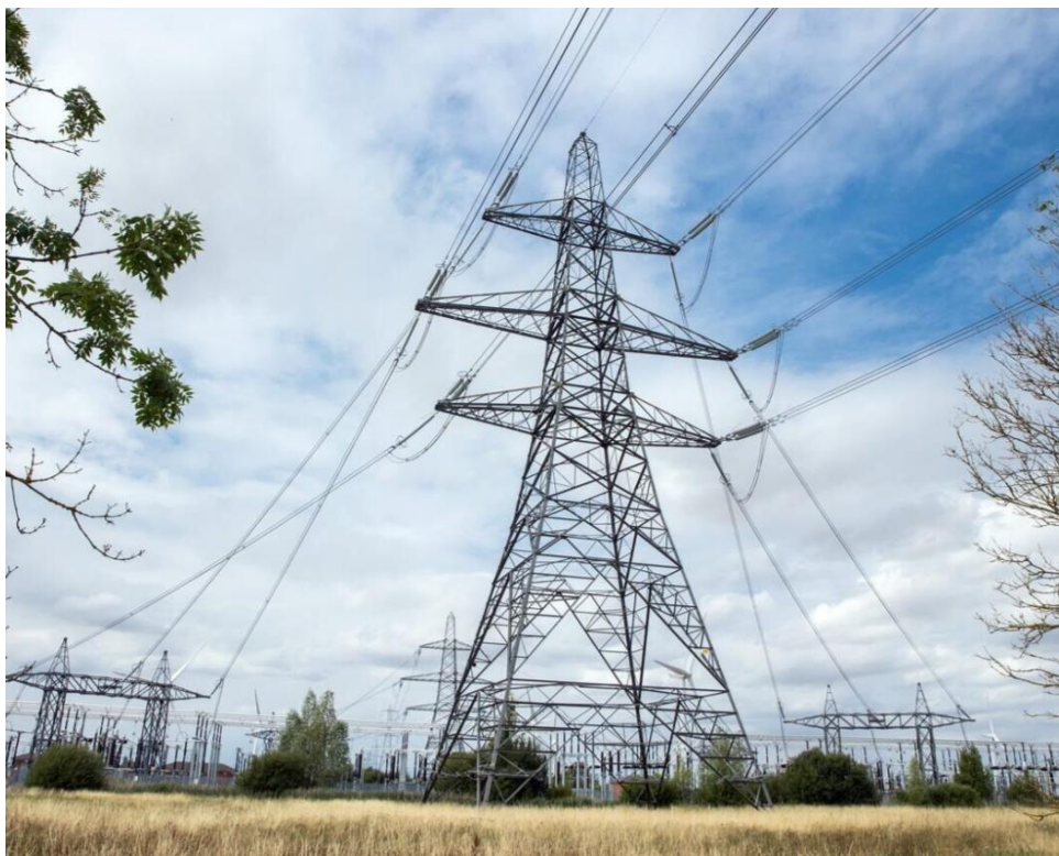
Image 5.13 Typical terminal lattice pylon 3
