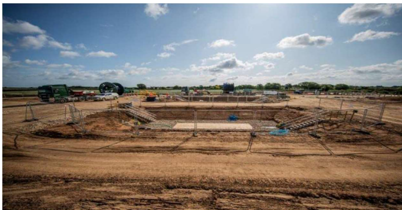
Plate 2-6 – A Typical Joint Cable Set Up
