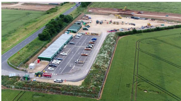
Plate 2-4 – Example Construction Compound Set Up
