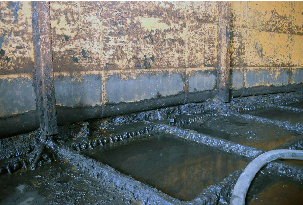
Plate 90: Outer section of floor
