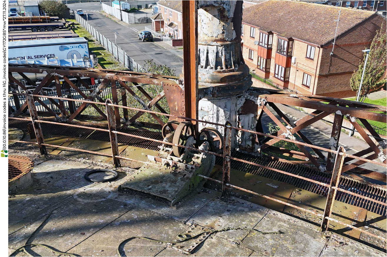
Plate 69: Detail of radial roller, taken from drone
