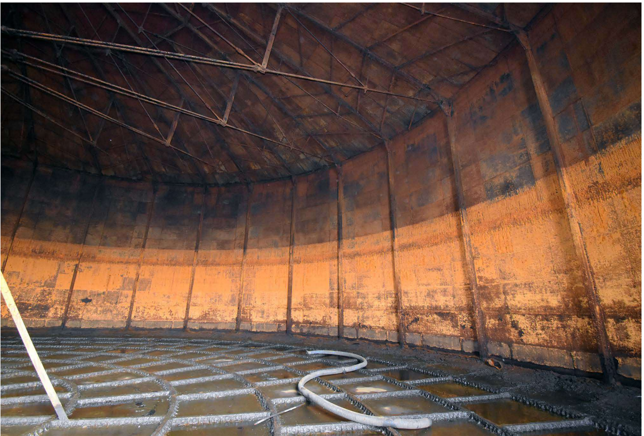
Plate 94: Typical section of wall (ie inner lift)
