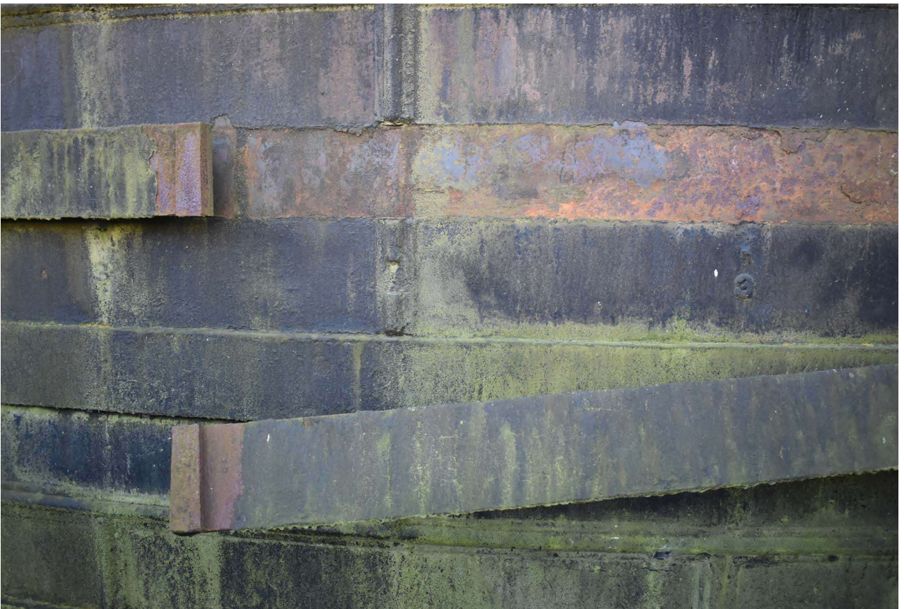
Plate 52: Bracing straps to side of holder
