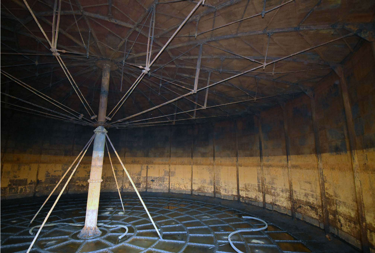
Plate 78: General view of interior
