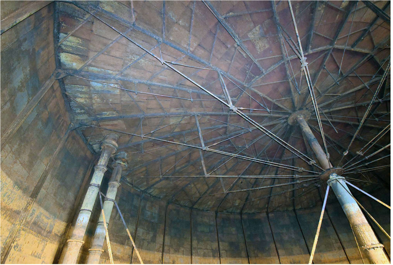
Plate 81: Radial roof structure
