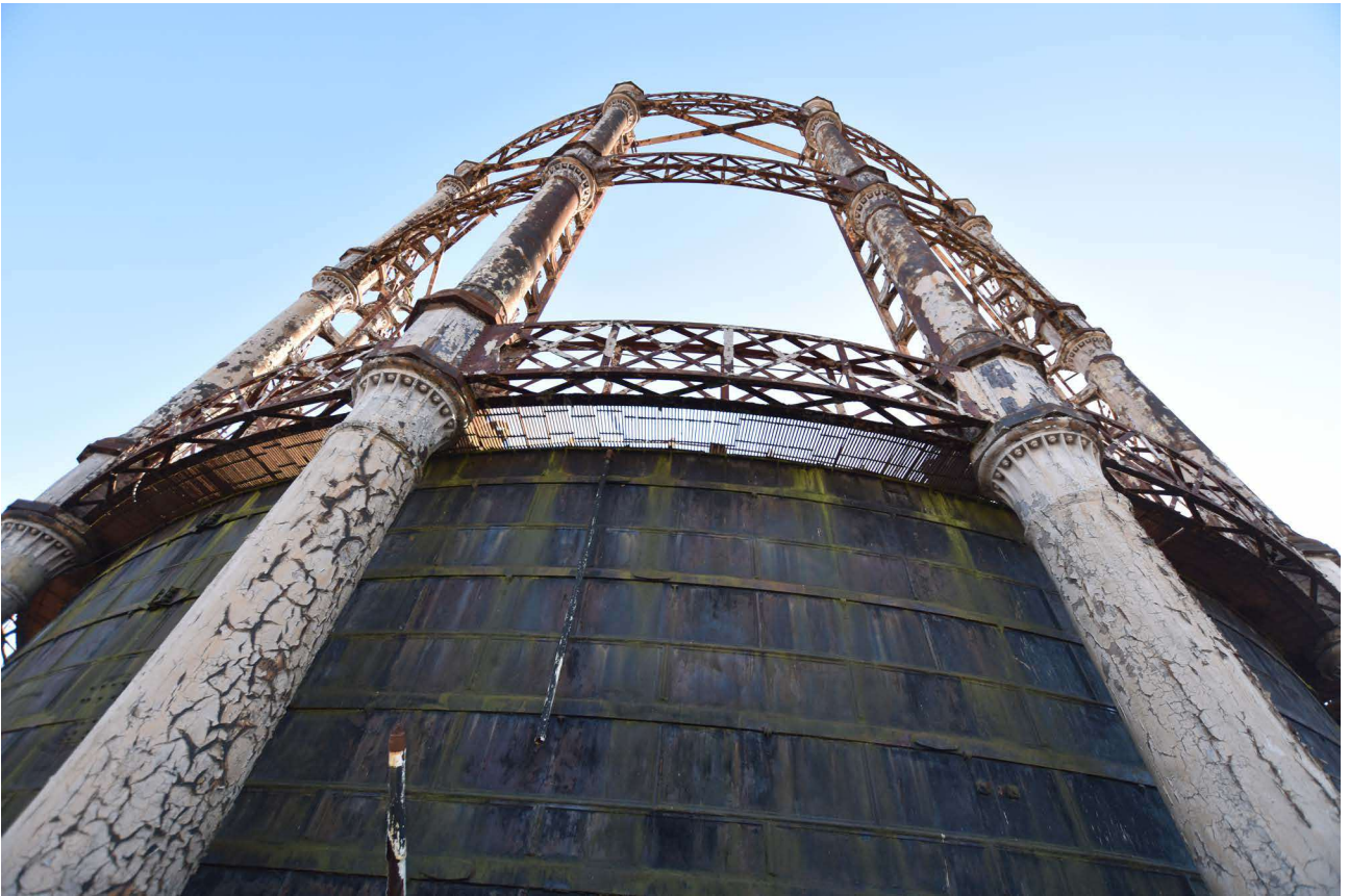
Plate 16: Vertical view showing tank and standards
