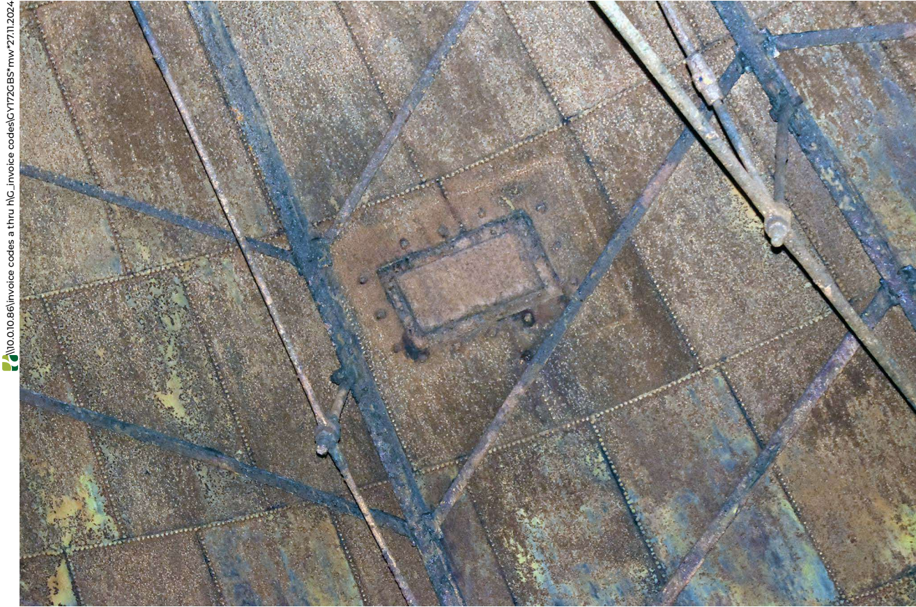
Plate 101: Detail of opening in crown
