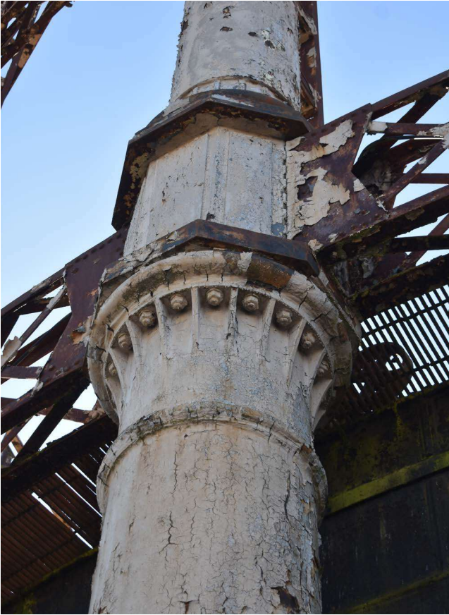
Plate 11: Detail of box junction
