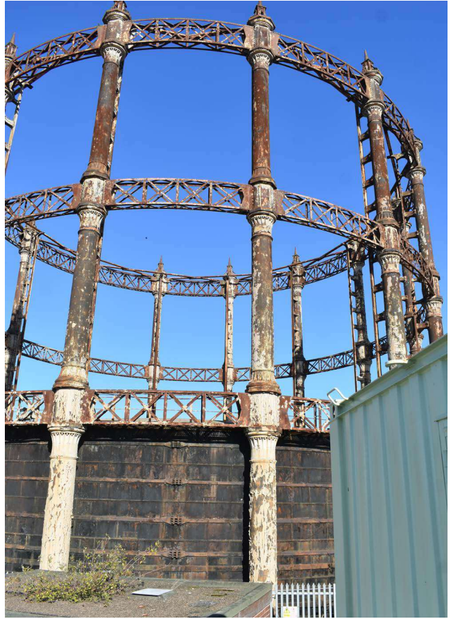
Plate 6: South side of gasholder
