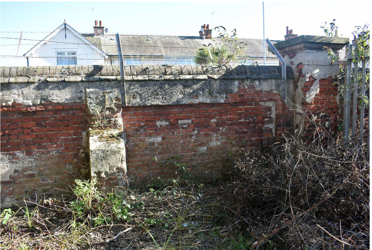
Plate 110: Section of brick wall to site boundary
