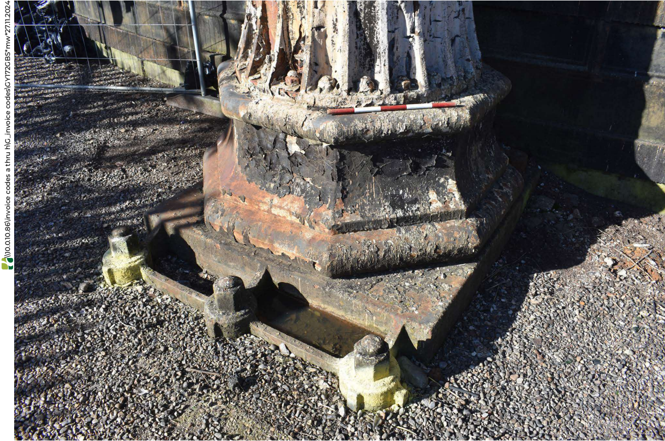
Plate 47: Example of column base
