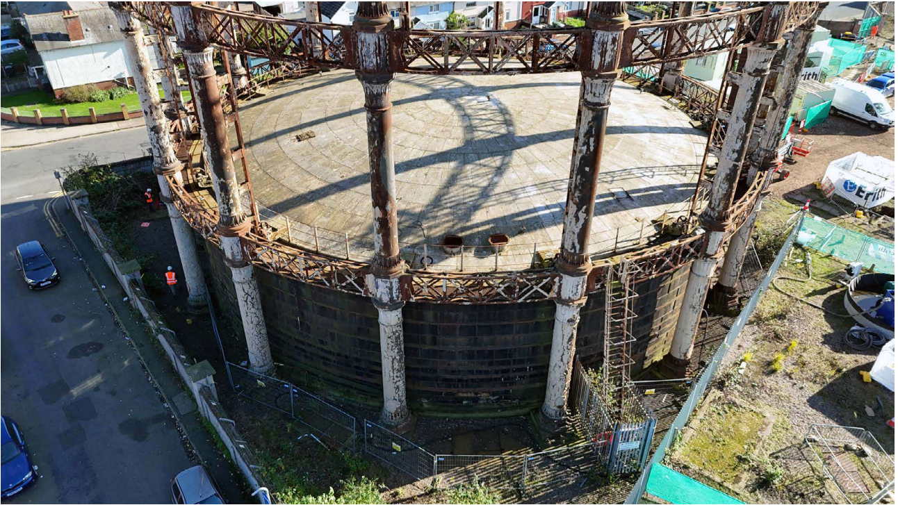
Plate 73: General view of tank, taken from drone
