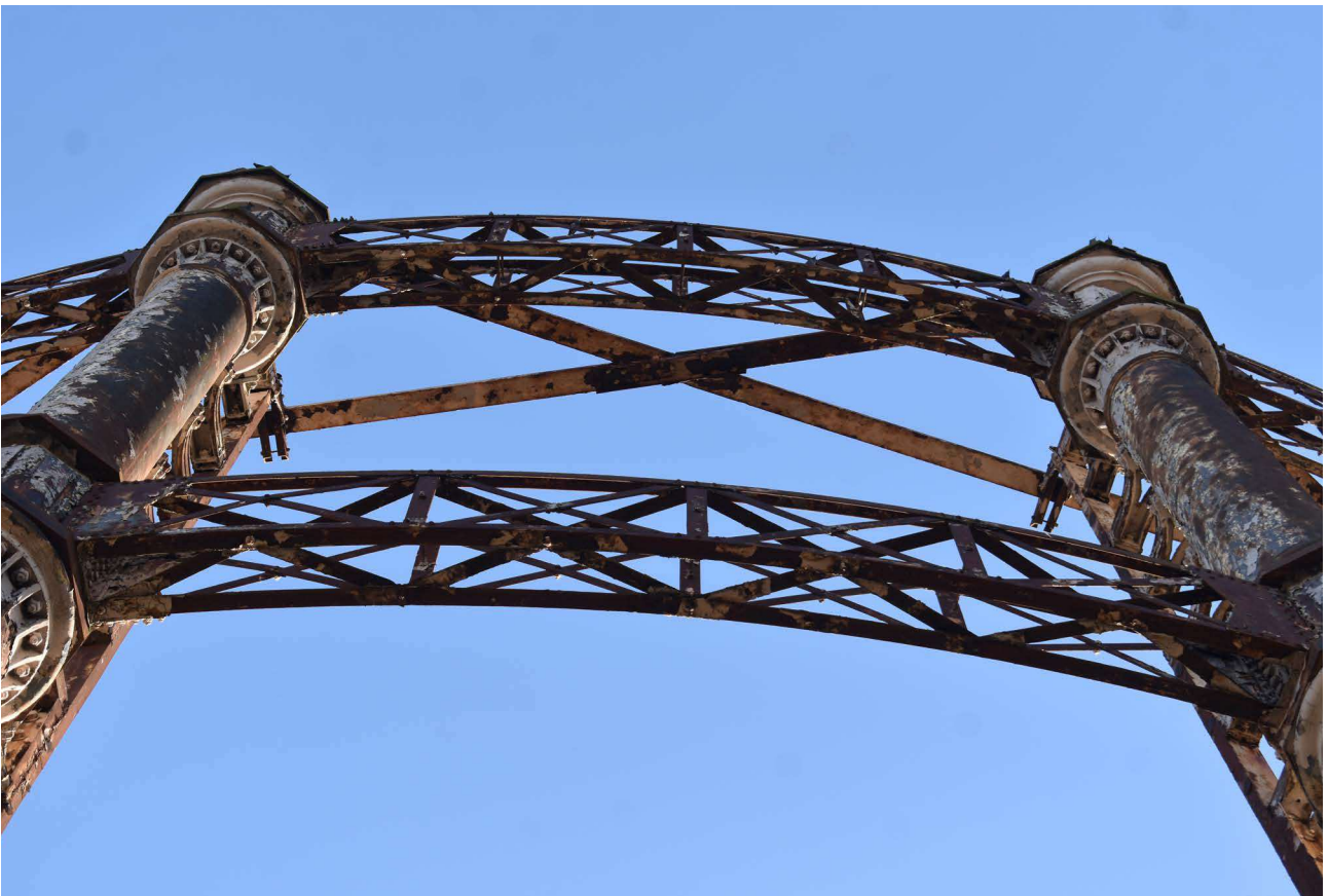
Plate 37: View showing curved girders
