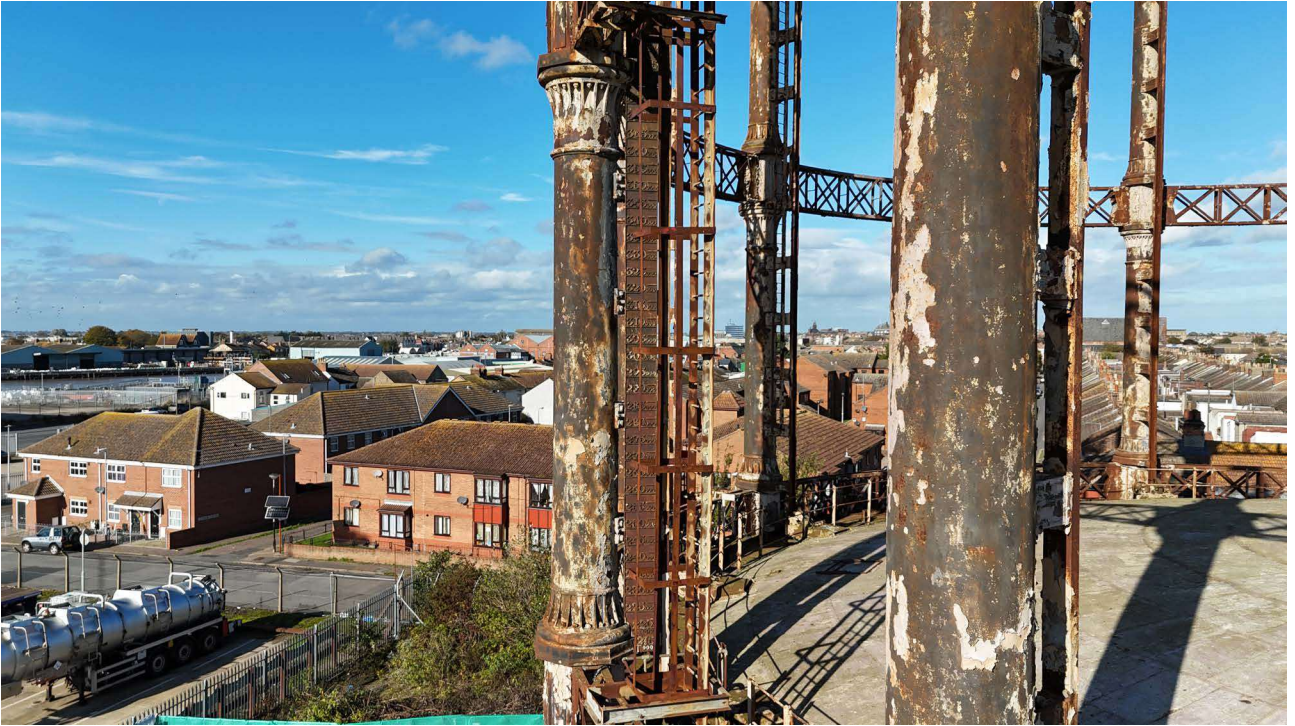
Plate 57: Detail of vertical gauge taken from drone
