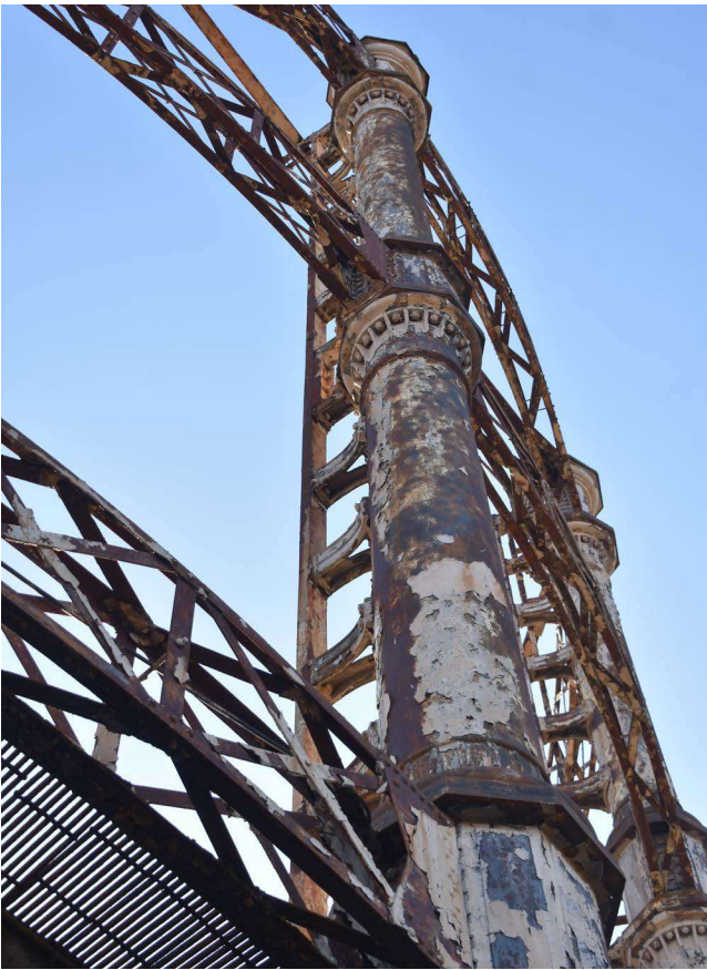
Plate 35: View of column
