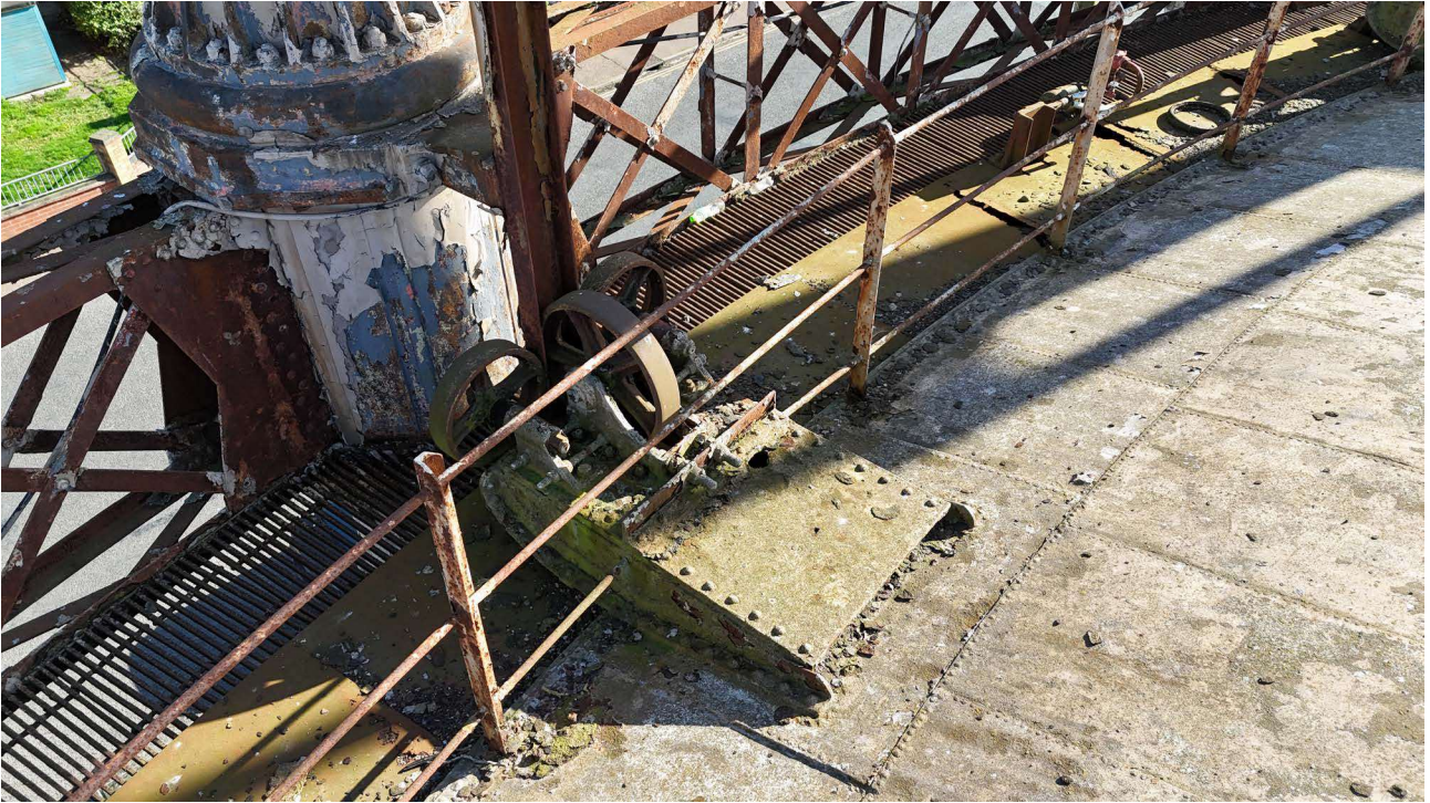
Plate 55: Detail of carriage roller taken from drone
