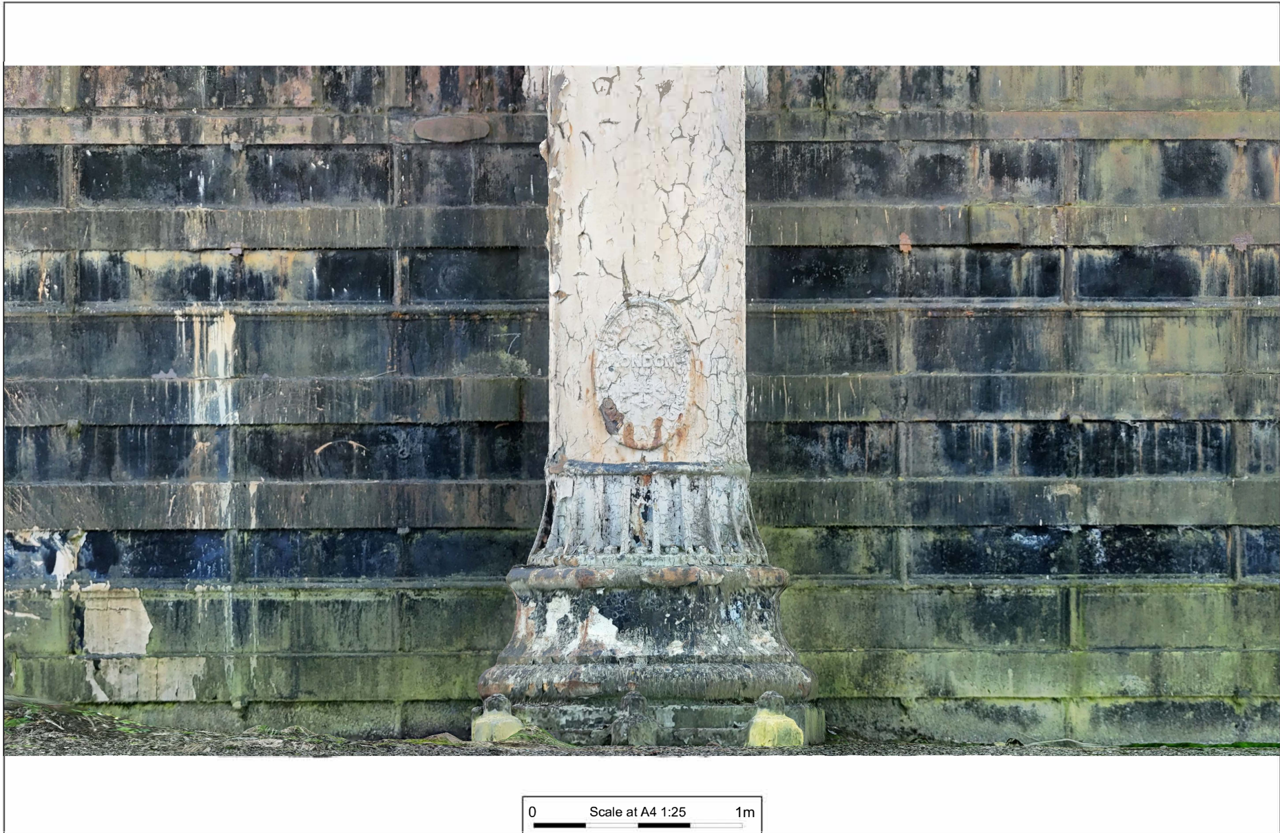
Figure 11: Image from digital 3D model showing column base and makers plate
