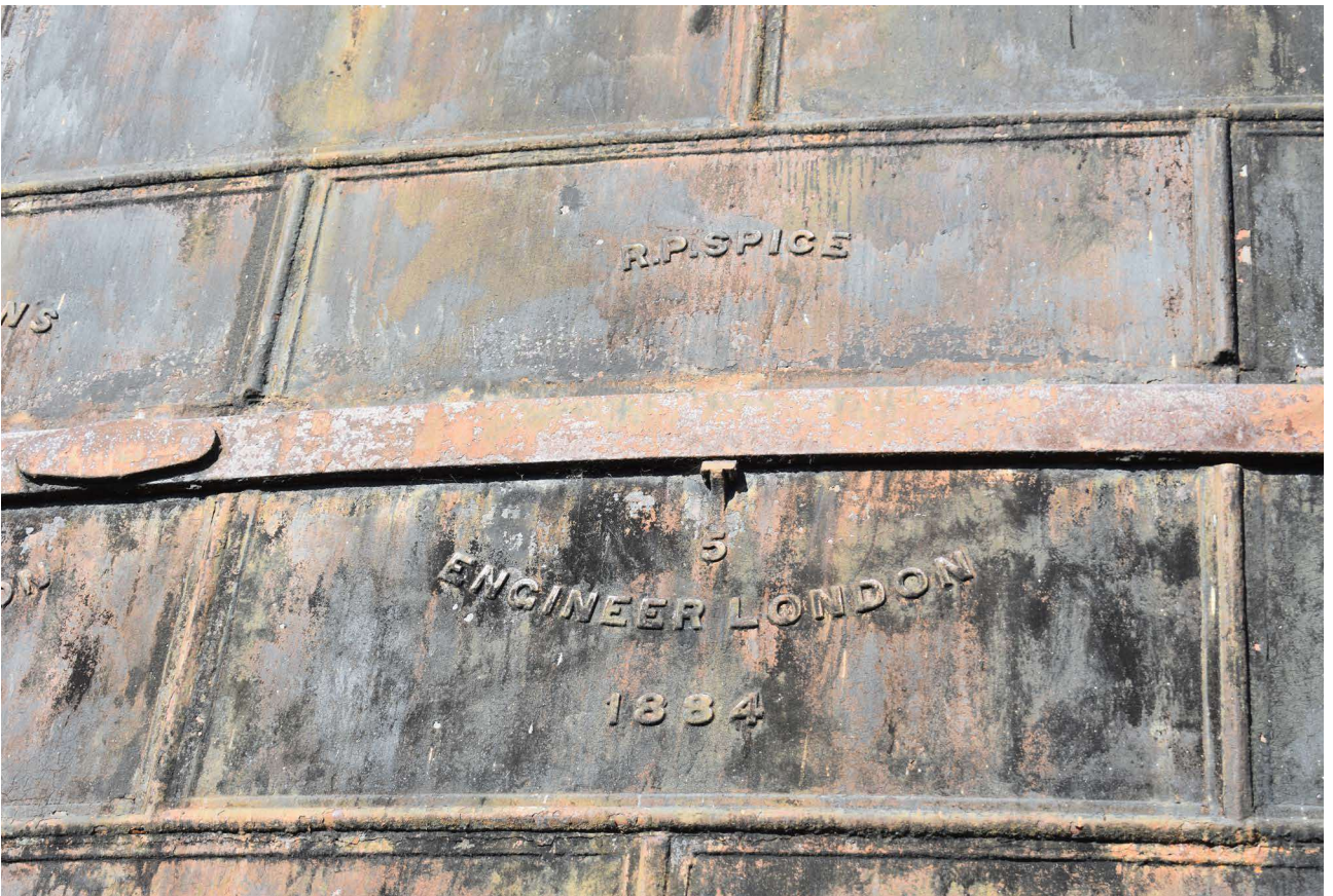
Plate 40: Side of tank with bracing
