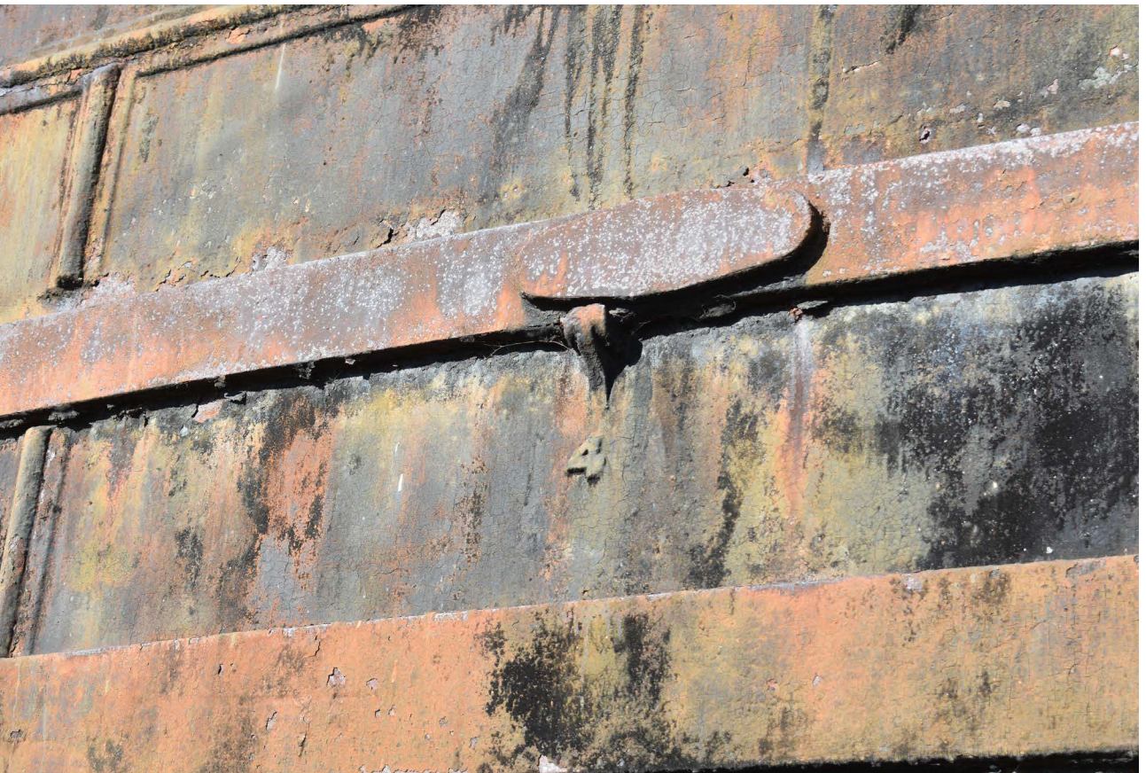
Plate 43: Bracing to side of tank
