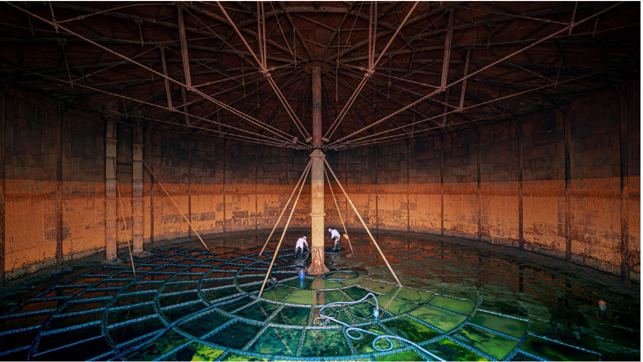
Plate 75: Interior during de-sludging (taken by Geoffrey Frost of Erith)
