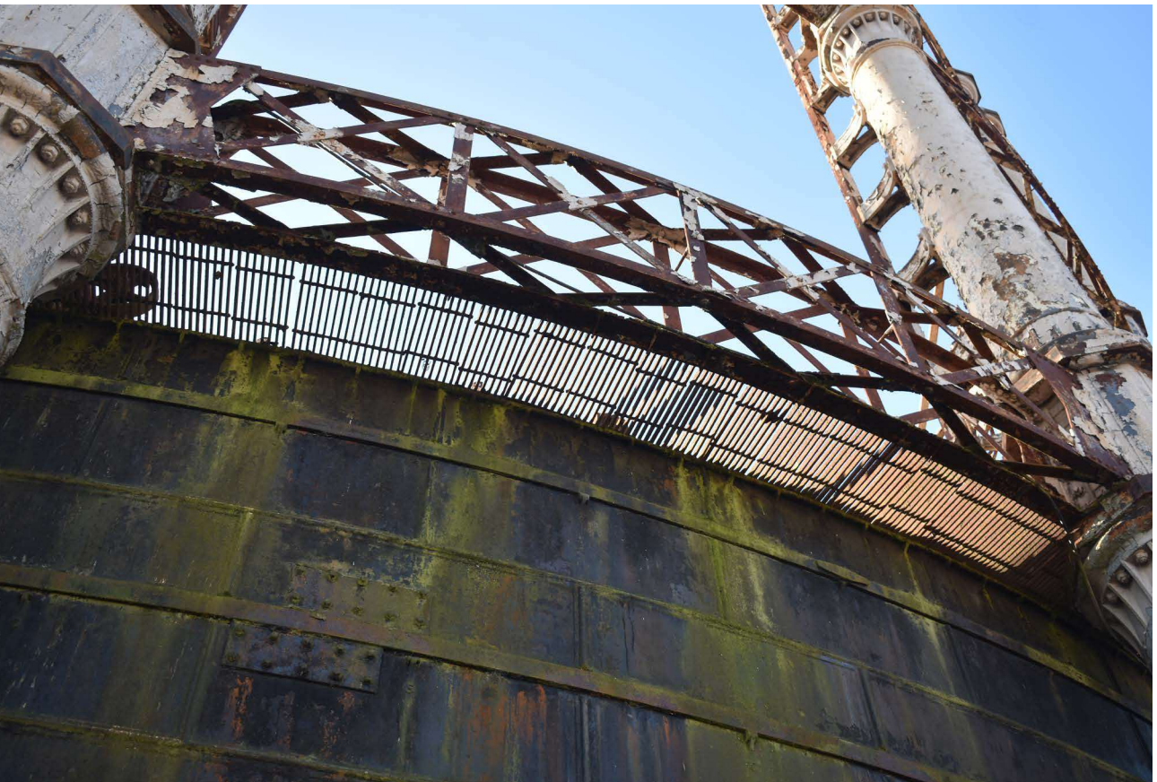
Plate 31: Example of walkway
