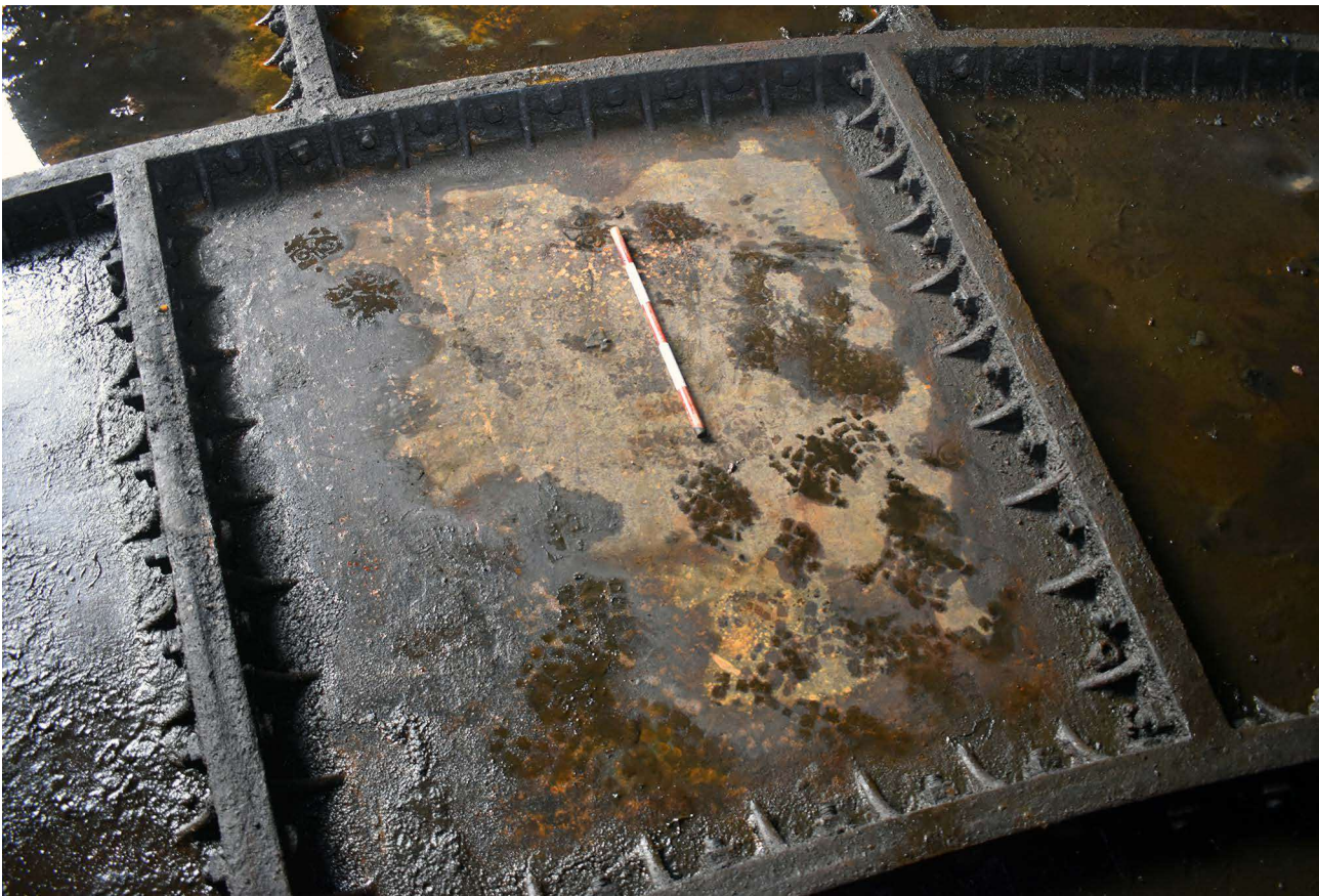
Plate 88: Detail of floor panel
