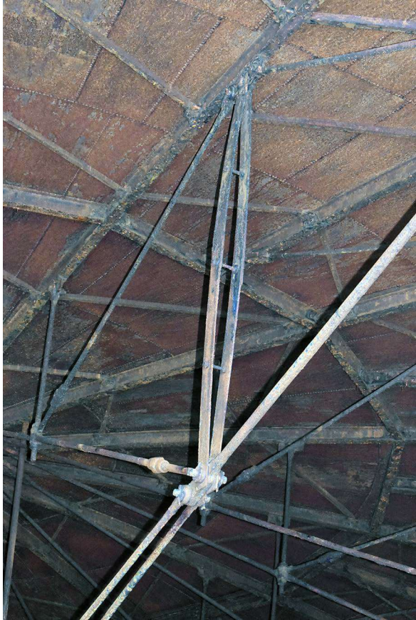
Plate 105: Detail of radial truss
