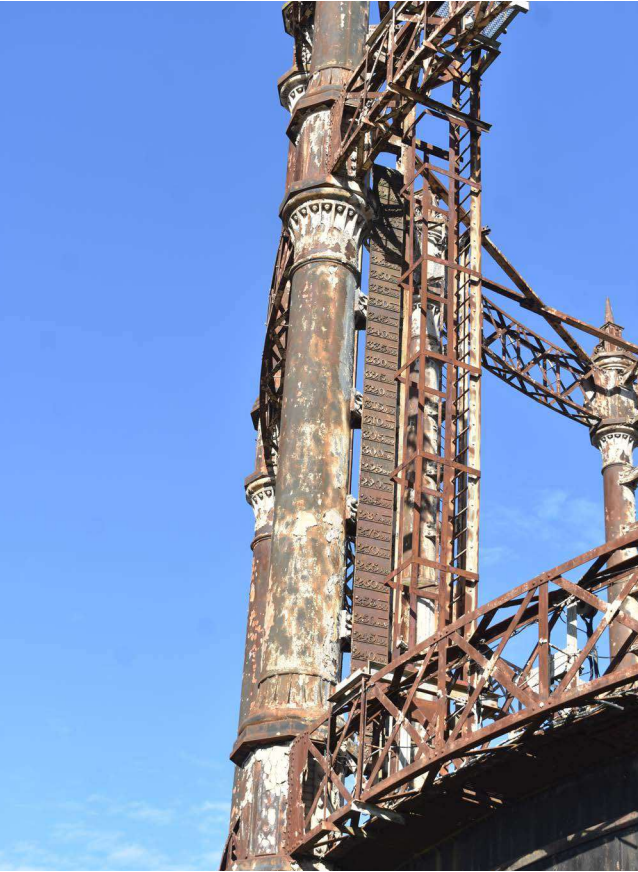
Plate 32: Detail of gas gauge
