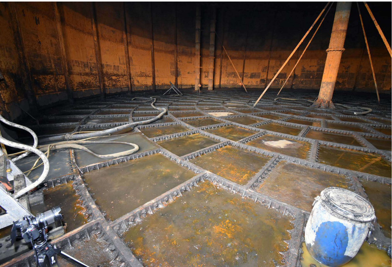
Plate 84: Floor structure within tank
