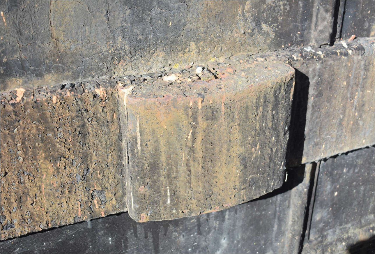
Plate 51: Brace lock to side of holder
