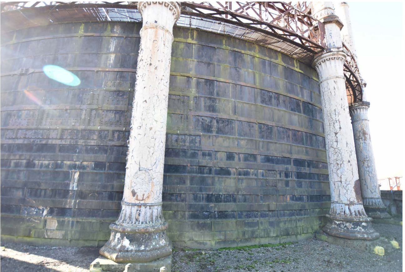
Plate 19: General view of tank
