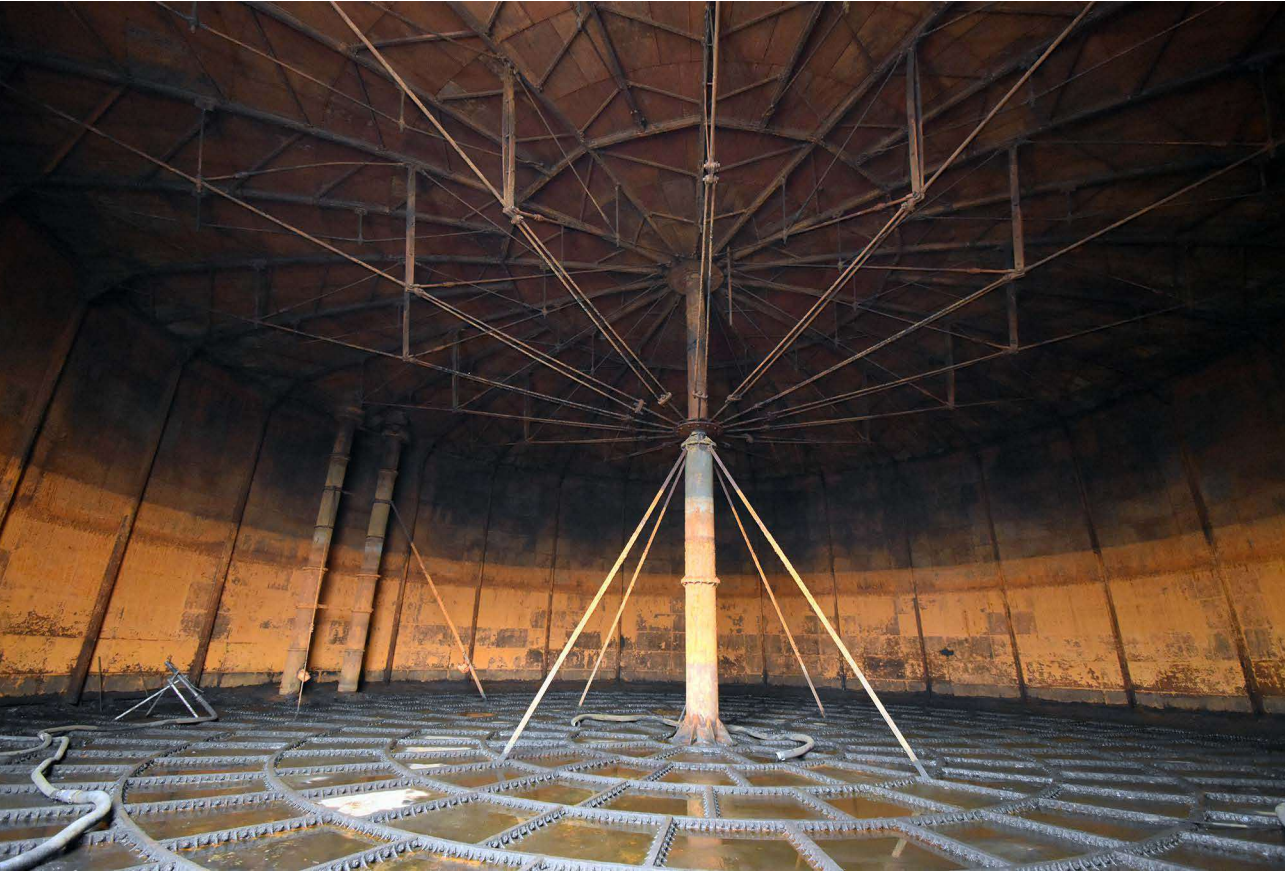
Plate 83: General view of interior
