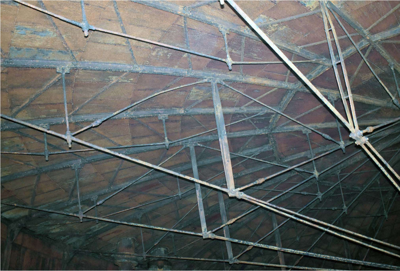
Plate 106: Detail of radial truss
