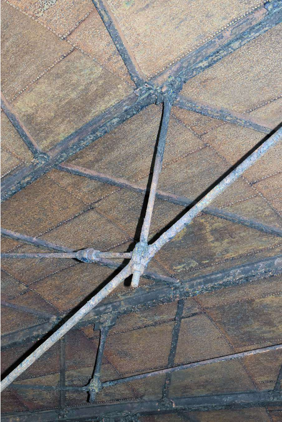
Plate 104: Detail of radial truss
