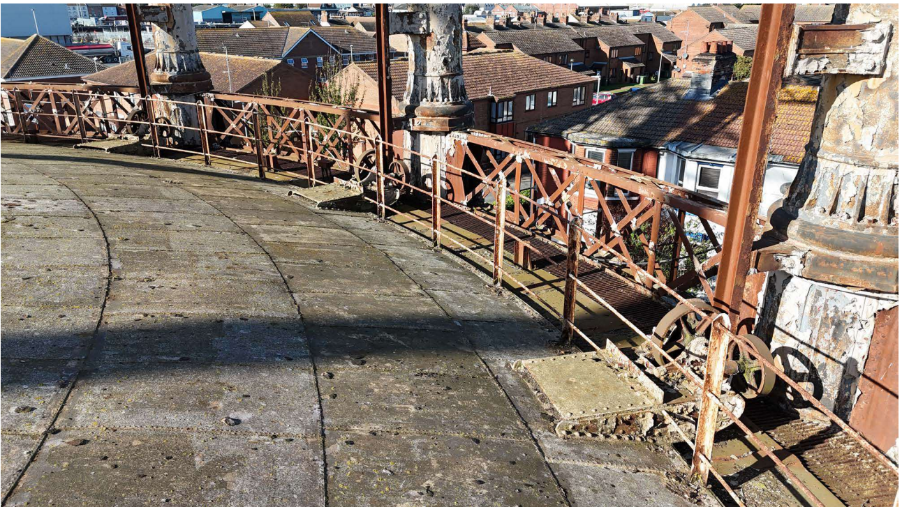
Plate 56: View on top of crown taken from drone
