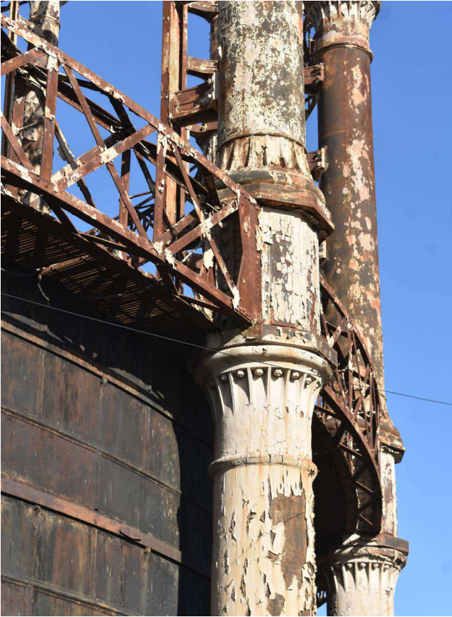
Plate 20: Detail of column head and junction box
