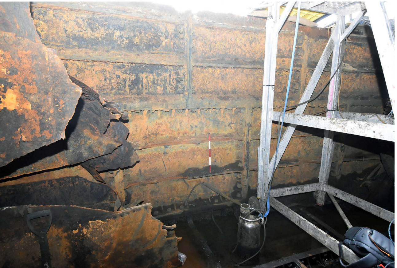
Plate 92: Exposed section of inner face of tank
