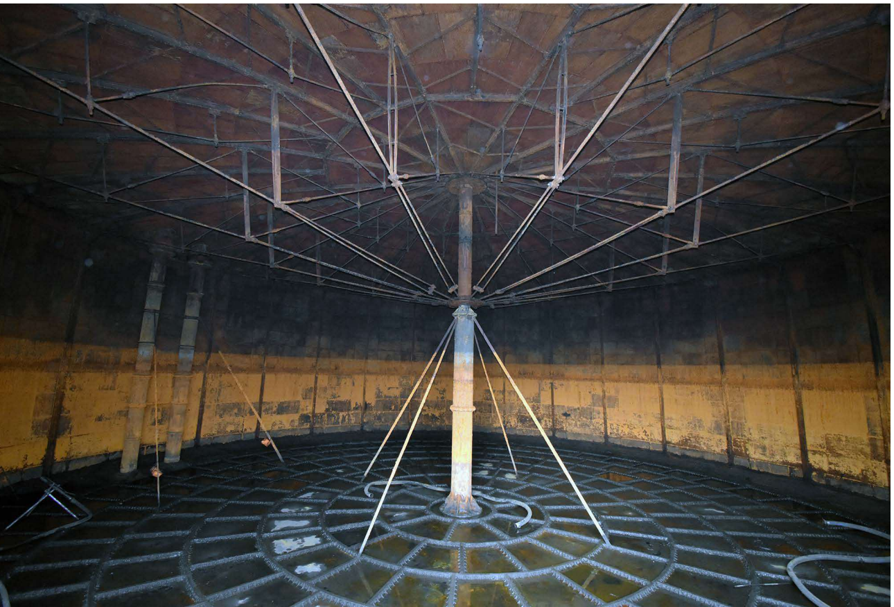
Plate 76: Interior following de-sludging
