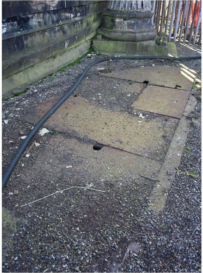
Plate 44: Bracing to side of tank Plate 45: Covers over pits to north-west side of tank
