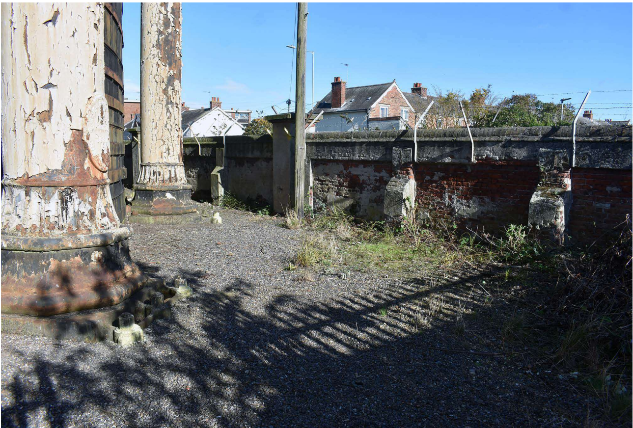
Plate 112: Brick site wall to east of holder
