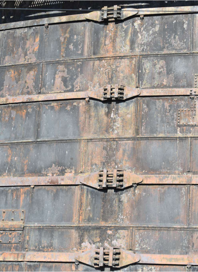
Plate 44: Bracing to side of tank Plate 45: Covers over pits to north-west side of tank
