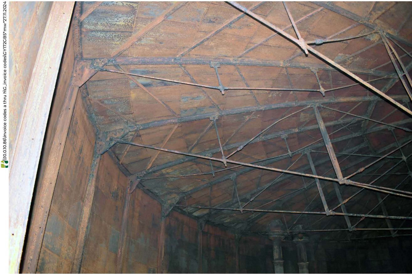
Plate 77: View of roof and wall
