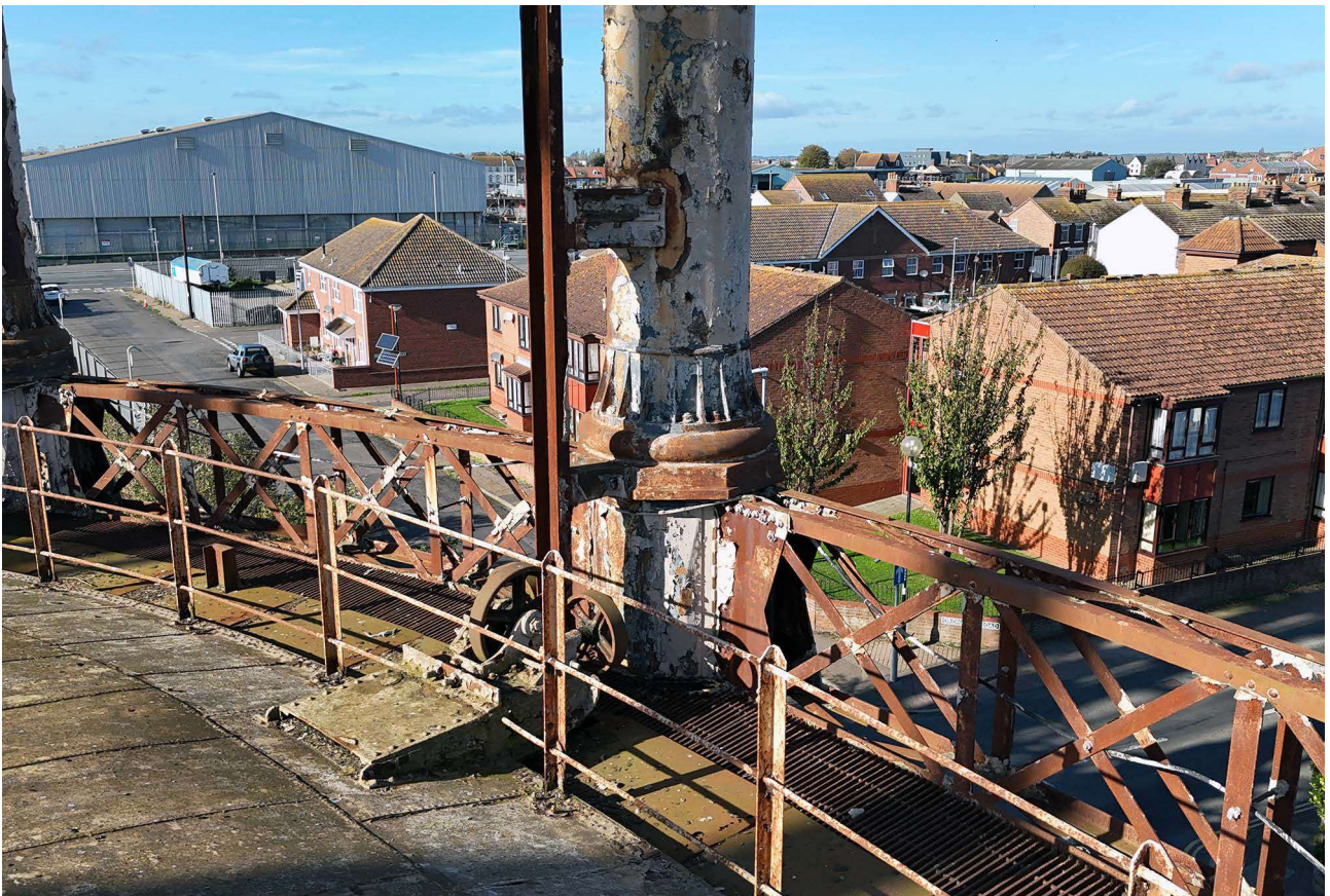
Plate 72: Detail of radial roller, taken from drone
