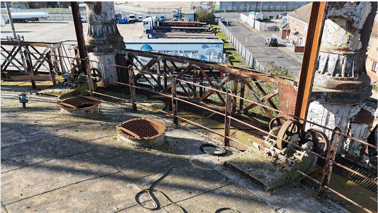
Plate 70: Detail on top of crown, showing inlet/outlet openings.
