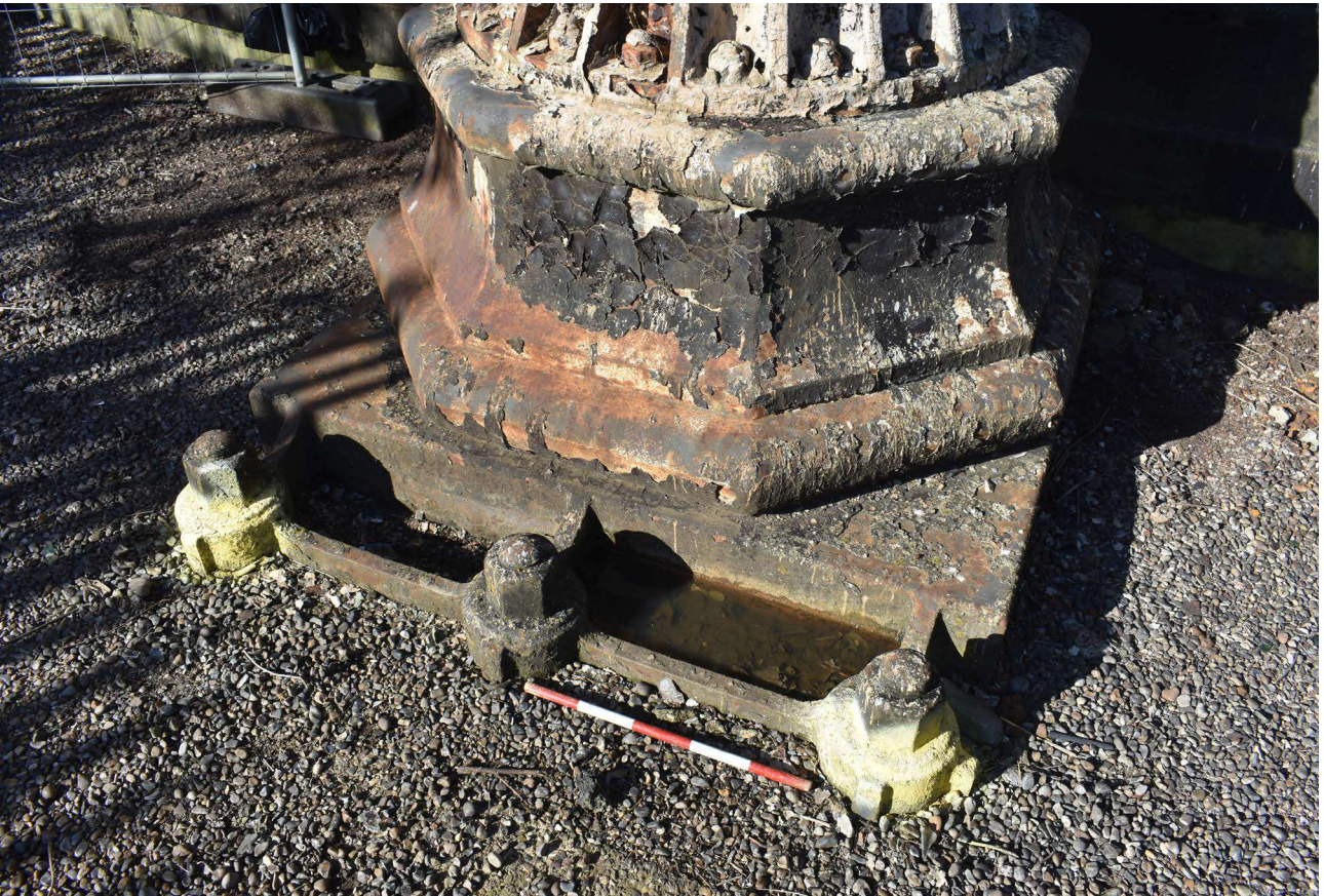
Plate 25: Example of column base
