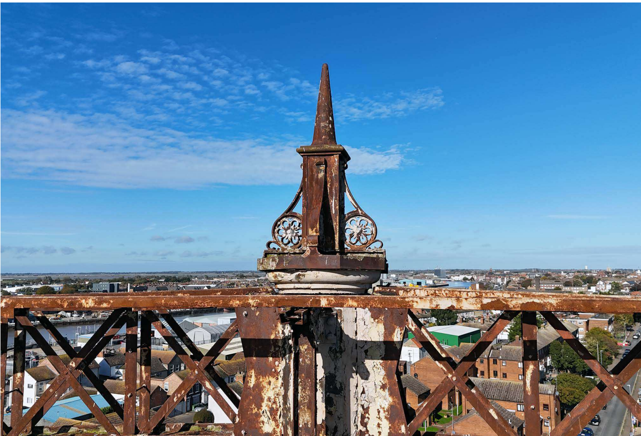
Plate 66: Finial to top of column, taken from drone
