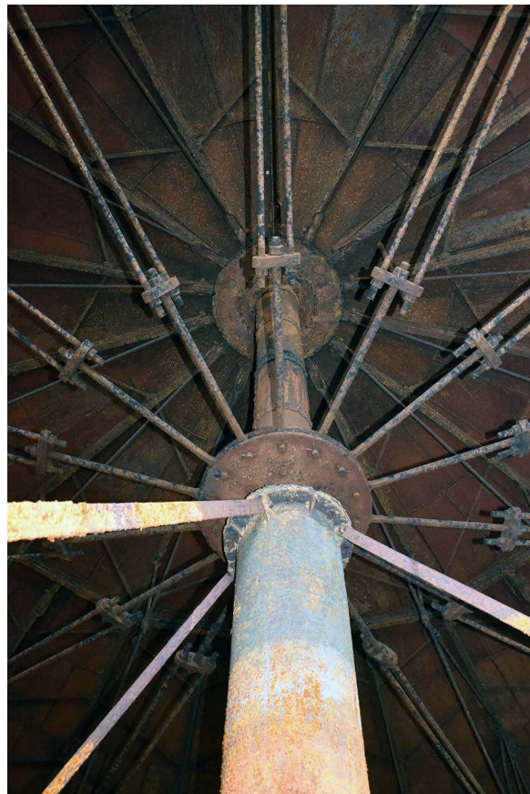
Plate 100: Detail of central shaft
