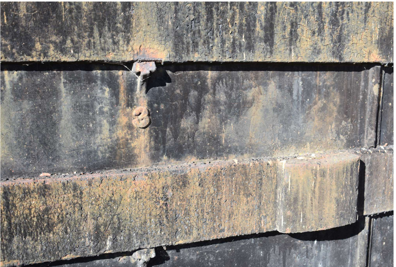
Plate 50: Brace lock to side of holder
