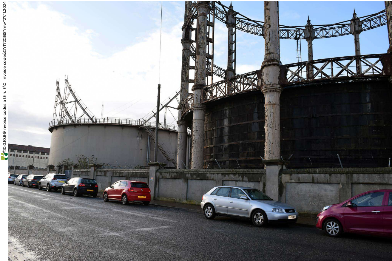
Plate 113: Holder 172 with now demolished Holder 173 to rear (taken Dec 2022)
