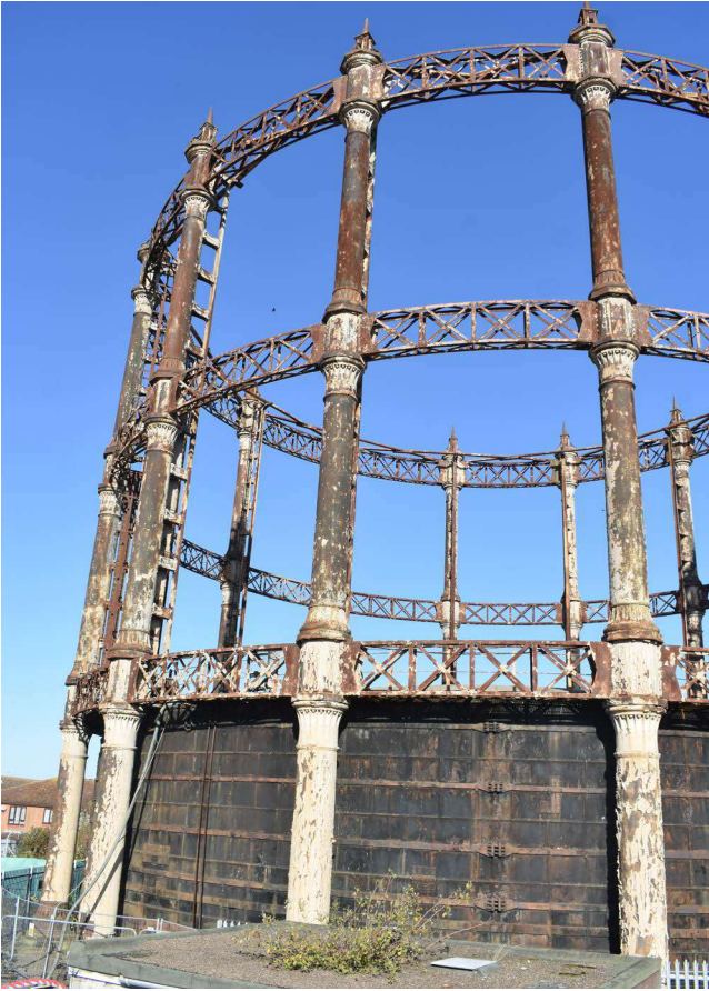
Plate 5: South side of gasholder
