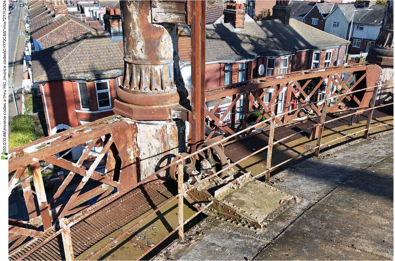
Plate 71: Detail of radial roller, taken from drone
