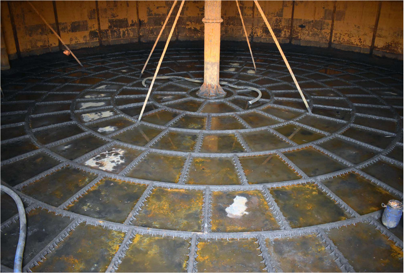
Plate 85: floor structure within tank
