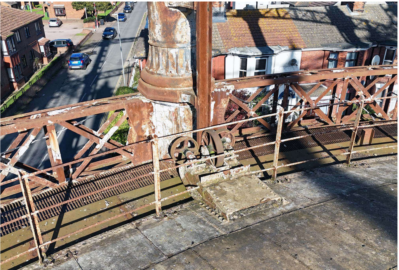
Plate 68: Detail of radial roller, taken from drone
