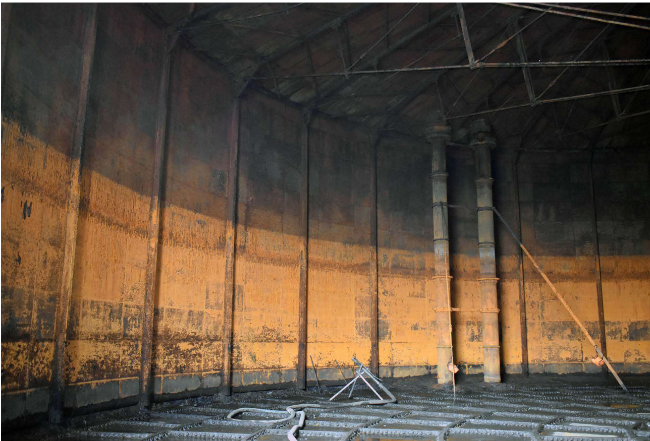
Plate 96: Section of wall within inlet/outlet pipes
