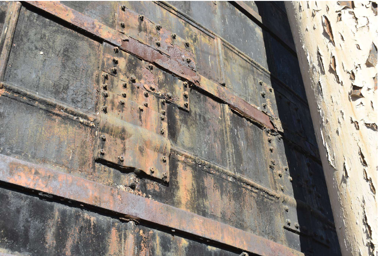
Plate 46: Remedial plates to side of holder
