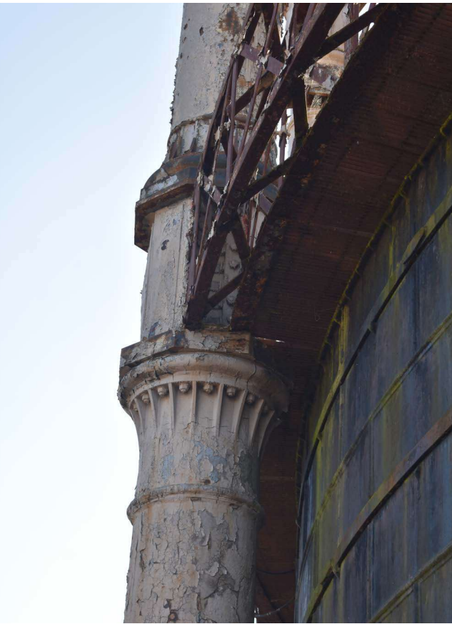
Plate 41: View of junction box
