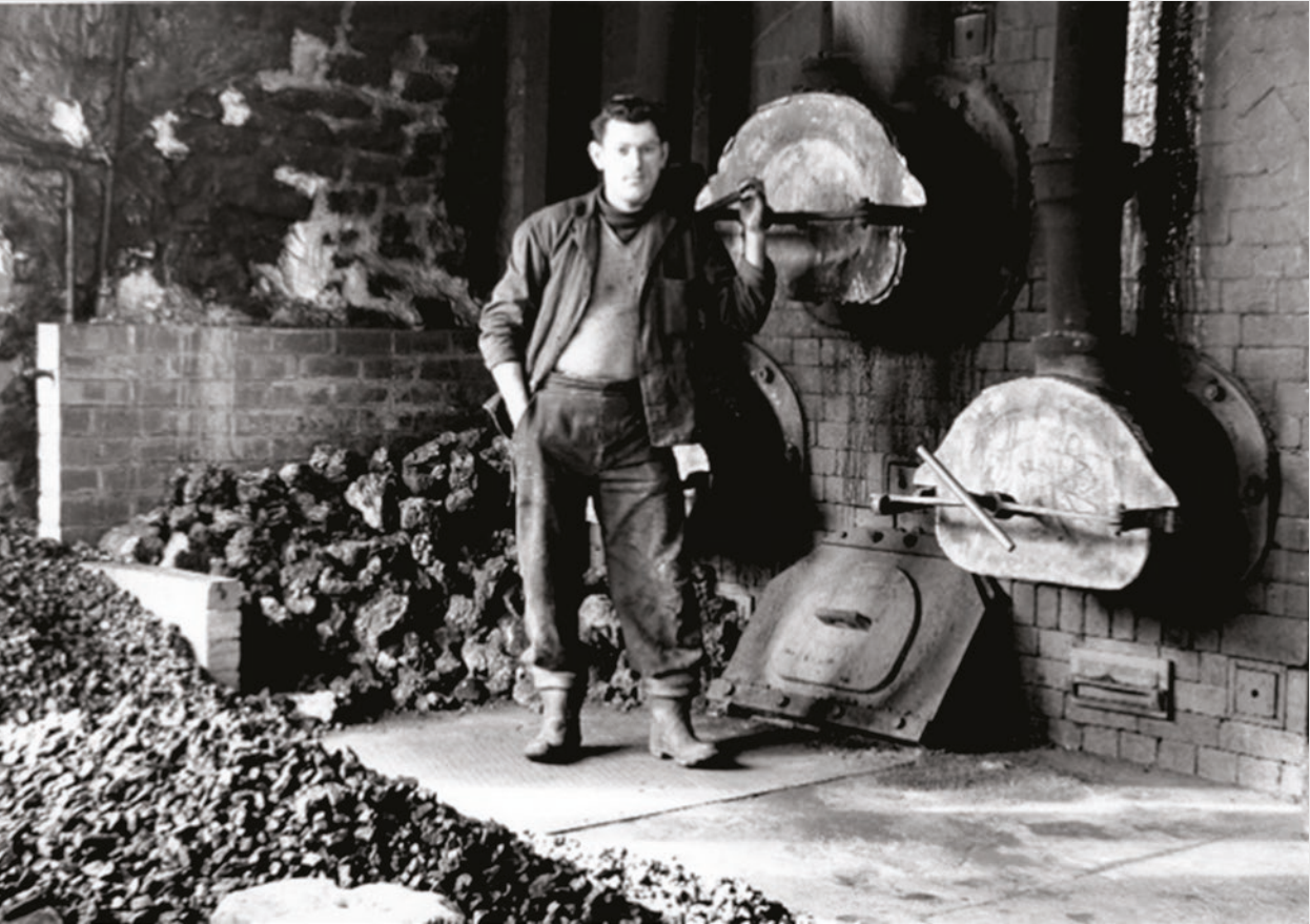
Figure 49. The stoker and horizontal retorts at the small former gasworks at Robin Hood's Bay, Yorkshire. Source: IGEM History Panel Archive.
