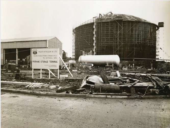
Figure 38. The propane storage tank built at Felixstowe, which supplied Cremorne Lane Gasworks at Norwich. Source: IGEN History Panel Archive.
