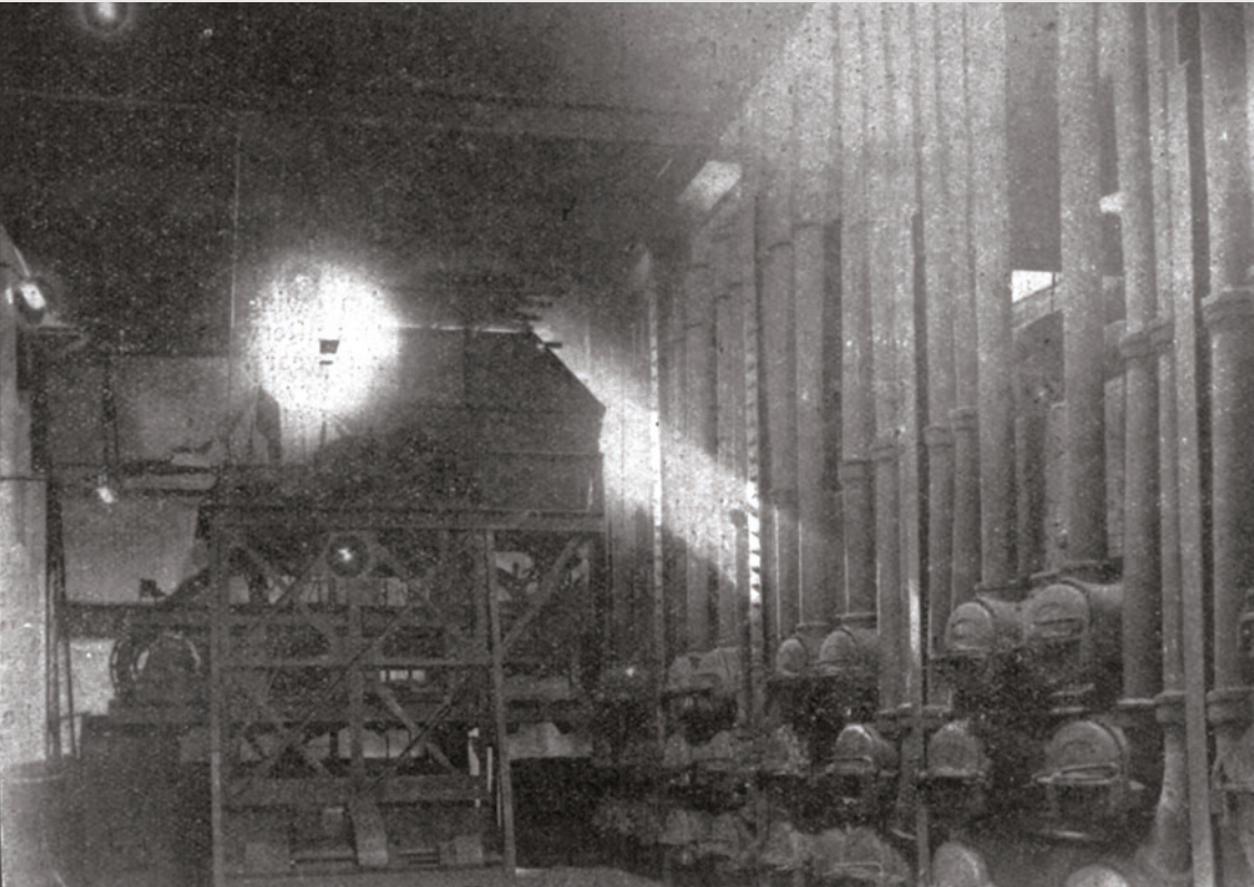
Figure 51. Guest-Gibbons charging and discharging machine at the Great Yarmouth Gasworks. Source: National Gas Archive.
