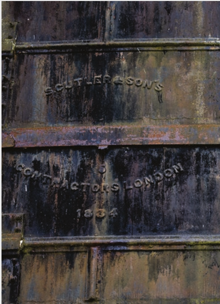
Figure 23. External detail of the tank wall showing the names of both R.P. Spice and Samuel Cutler and Sons, with the date 1884. Source: Jam Butty Photography and Video and IPB Communications.
