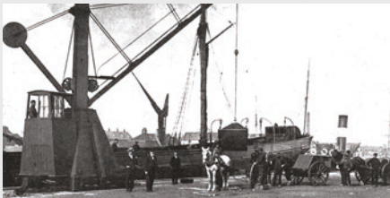
Figure 25 (above). The hydraulic crane in action, unloading skips onto framework carts. Source: National Gas Archive.
