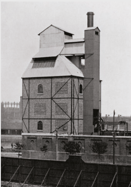
Figure 16. The vertical retort house installed at the Gorleston Gasworks in 1929 by Woodall-Duckham. Source: IGEN History Panel Archive.
