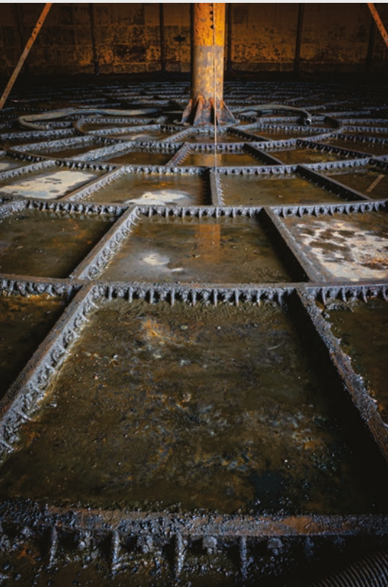
Figure 19. The cast iron flanged plates on the base of the tanks. Source: Mike Glyde.
