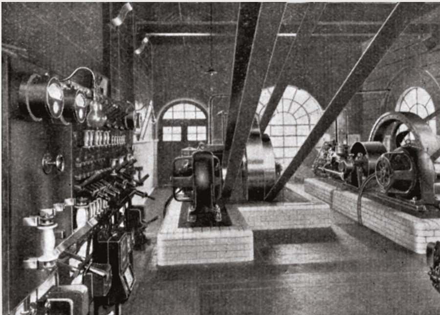
Figure 28. Powerplant installed at the Great Yarmouth Gasworks. Source: National Gas Archive.
