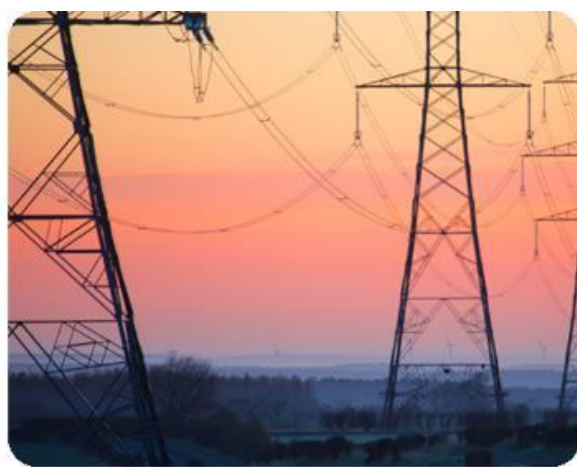
National Grid Pylons and Overhead Lines
