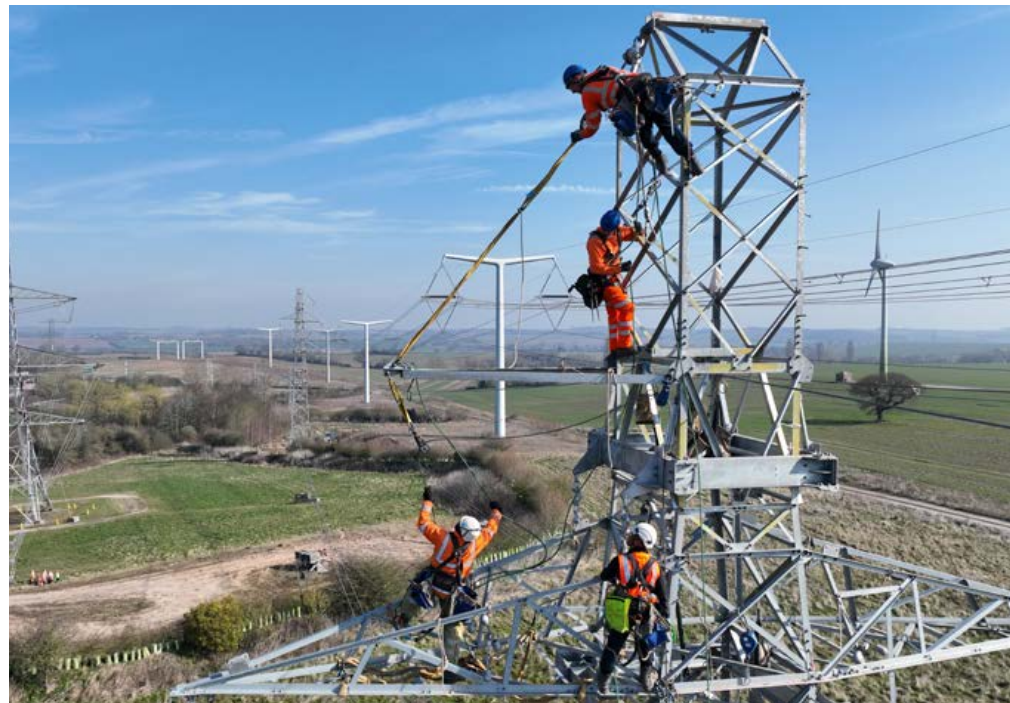
RICAs being constructed at Eakring.
