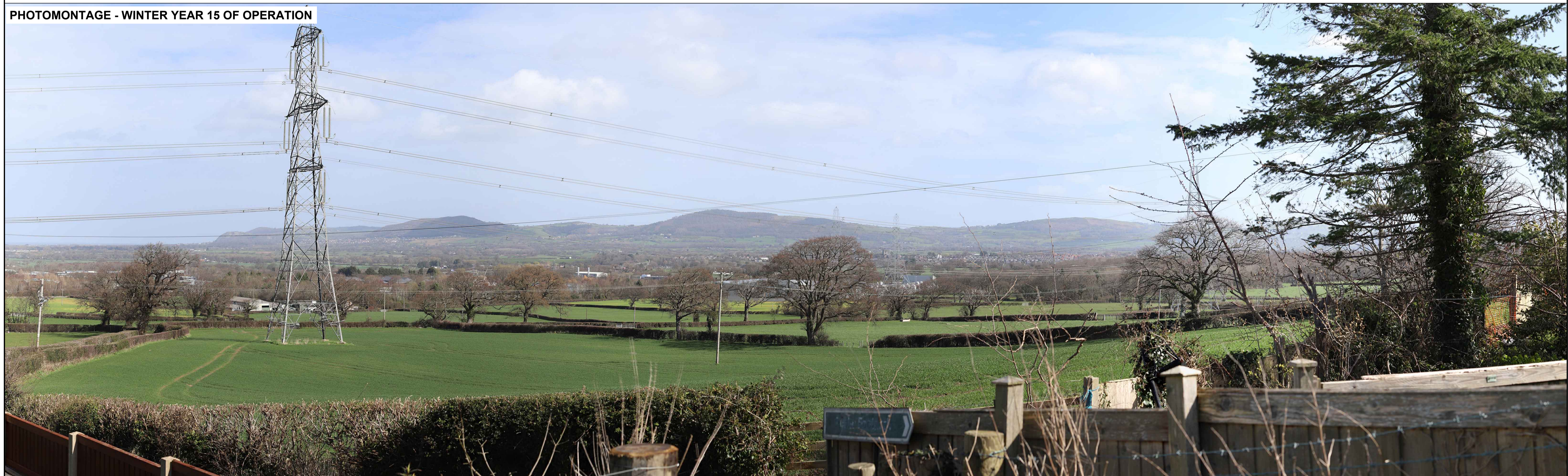
VIEWPOINT 22: View looking north east from footpath towards Substation
