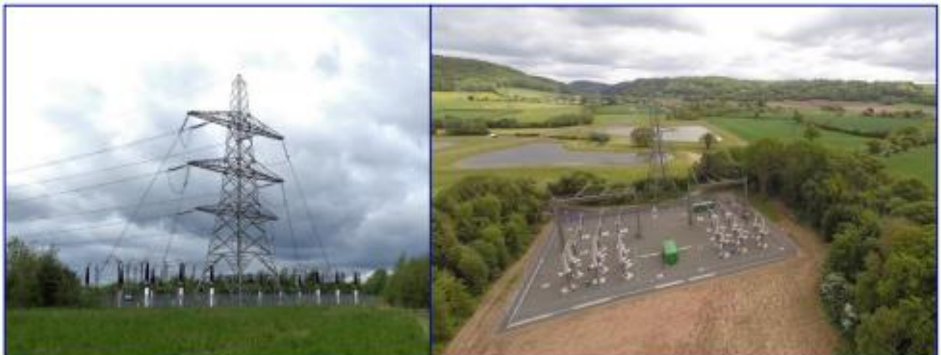
Figure 2-6 — Example 400kV sealing end compounds with terminal pylons
