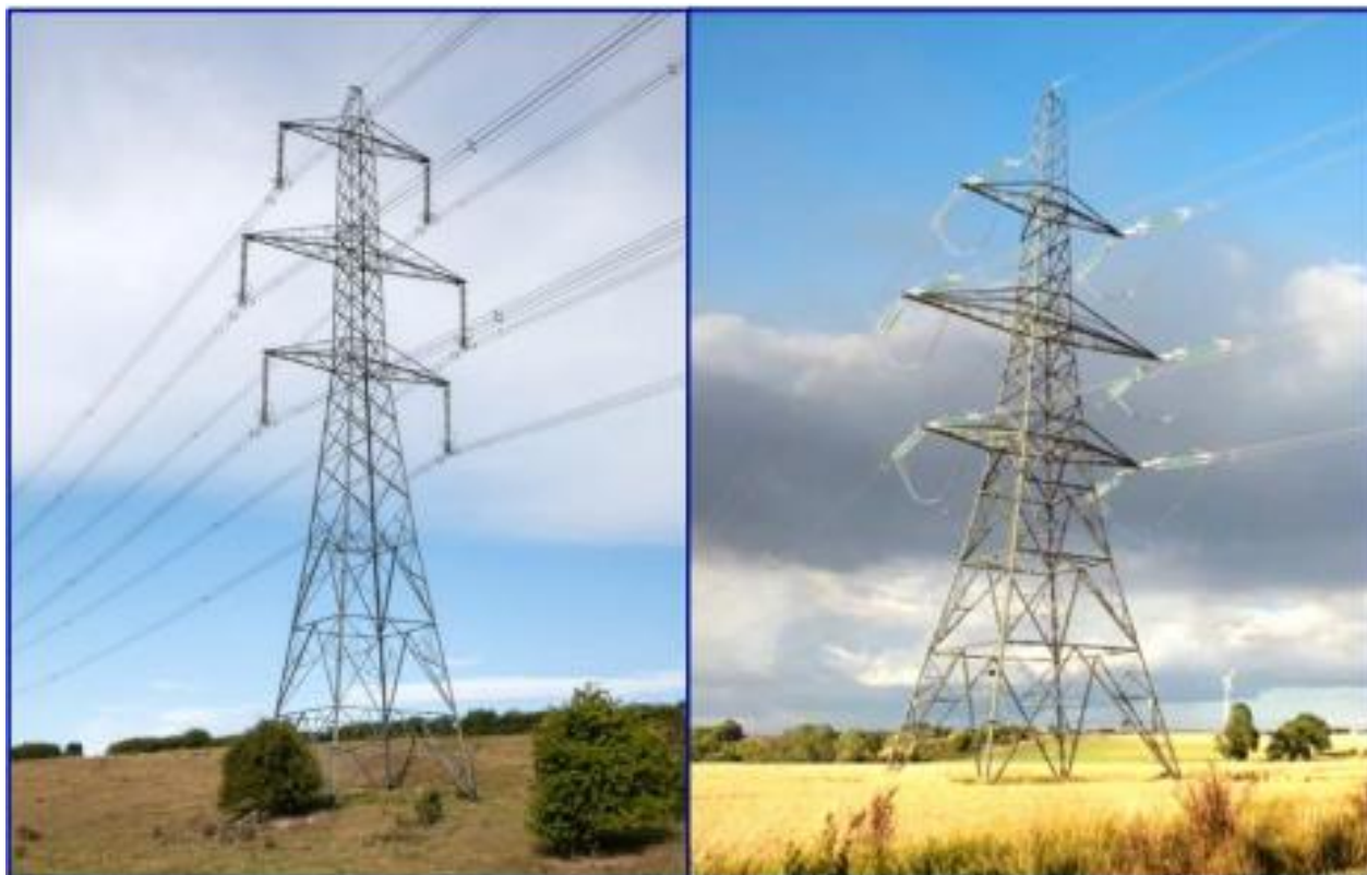
Figure 2-2 — Suspension Pylon (Left) and Angle Pylon (Right)
