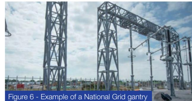
Figure 6 - Example of a National Grid gantry
