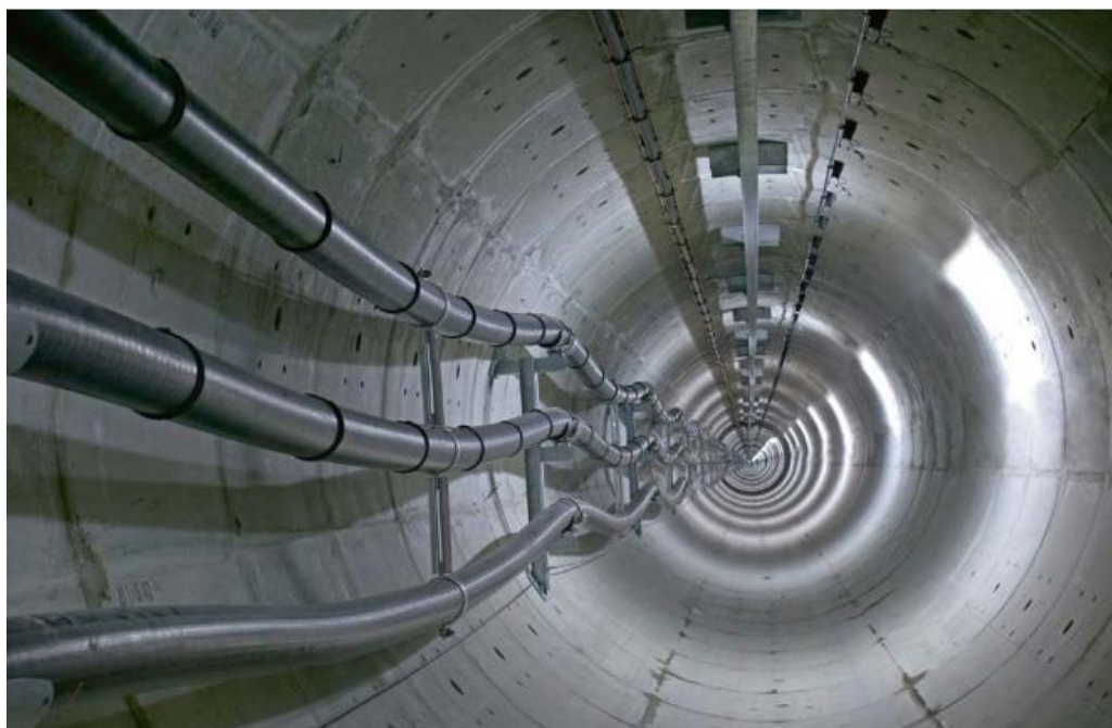
Figure 3-1: Example of XLPE Cables installed in a deep bored tunnel
