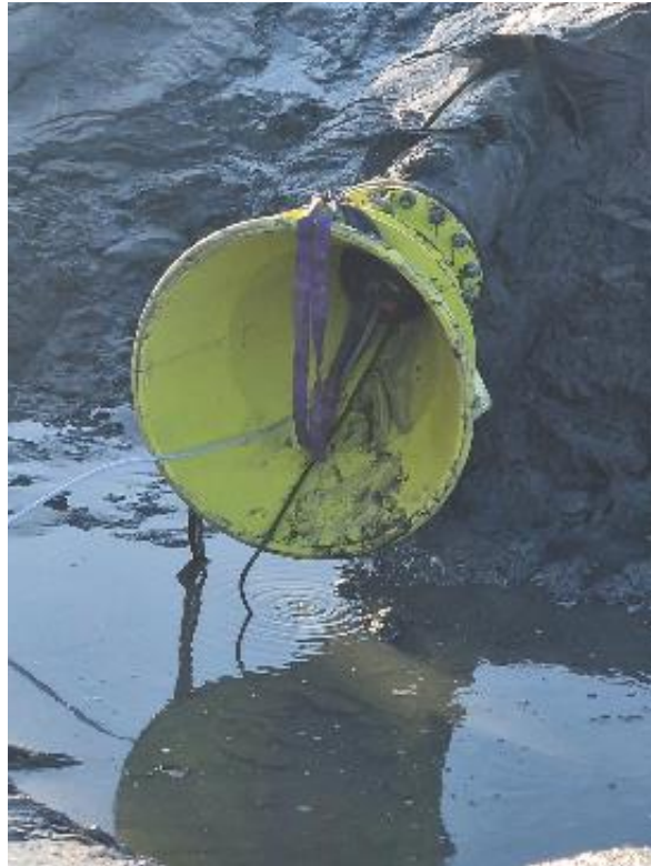
Plate 4-14: Example of a marine bell mouth
