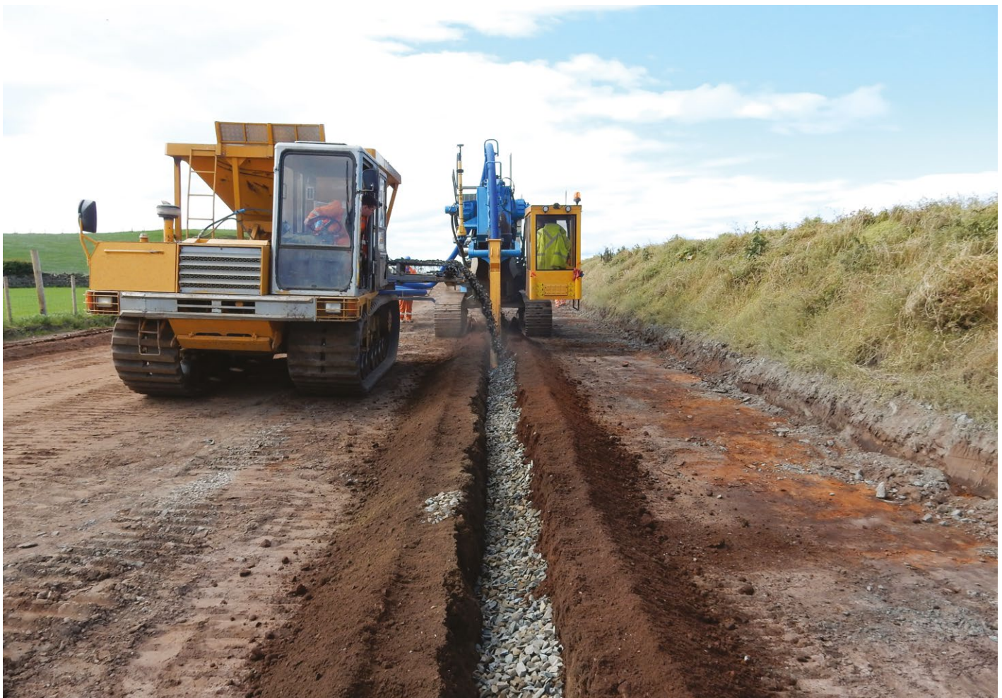
Example installation of pre-construction drainage system along High Voltage Direct Current project
