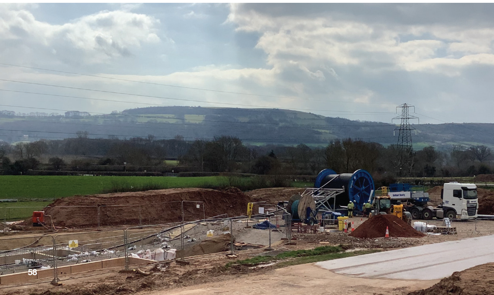
Figure 28 – The ducted method of cable laying
