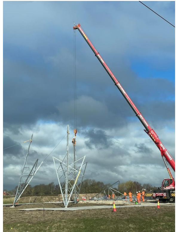
Image caption: Crane in use at Moor Monkton to build a pylon.
