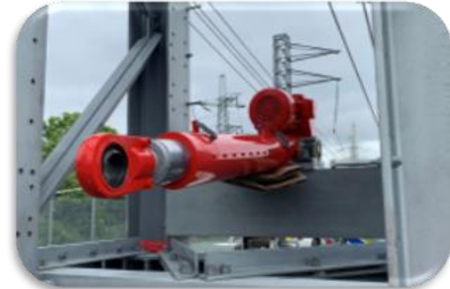
300 kN actuator for conductor tensioning
