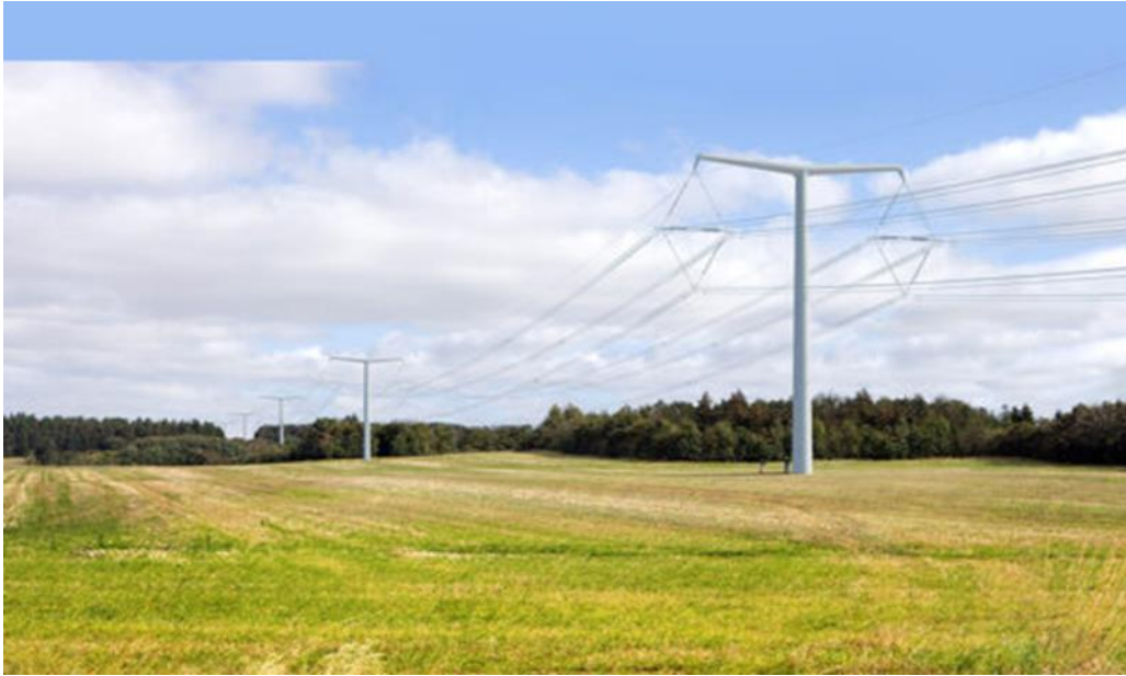
Figure C.2 – The T pylon
