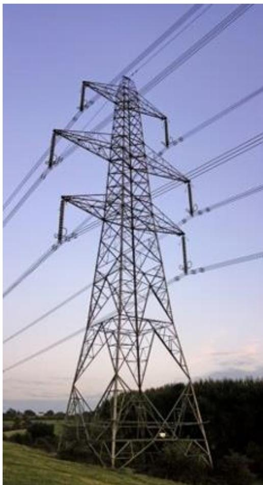
Image 4.6 - Typical tension/angle lattice pylon
