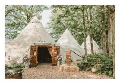
The proposed tipi structures (as above) comprise a timber frame construction with canvas sheet covering to provide enclosure. These units are demountable for cleaning and maintenance purposes and can be stored out of season for protection from the worst of the weather. They are erected on a timber frame base on compacted hard standing and pad foundations to specific areas.
