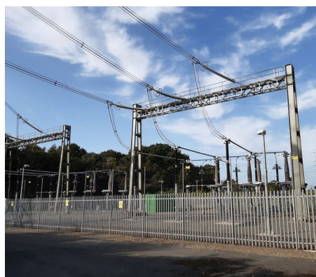
Cable sealing end compound
