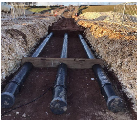
Constructing underground cable
