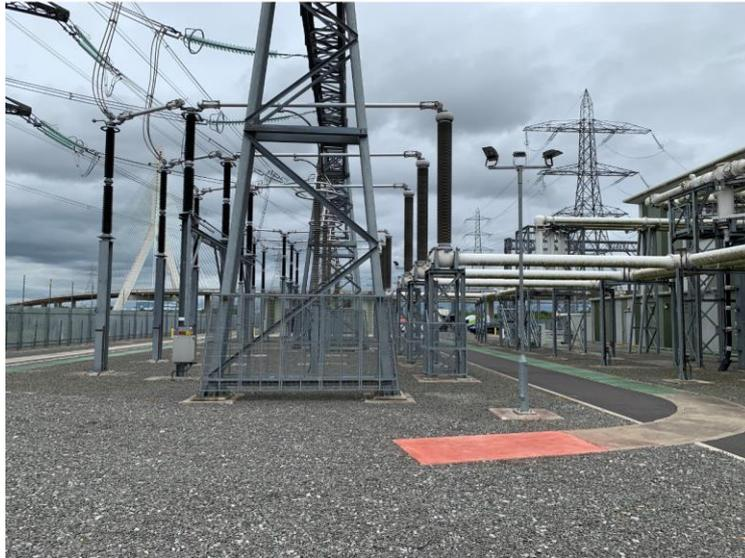
Photo 3. Illustrative view of the Substation showing GIB & AIS equipment connecting to a Gantry and OHL.
