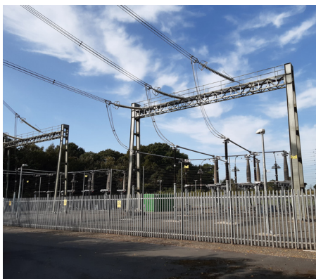
Cable sealing end compound
