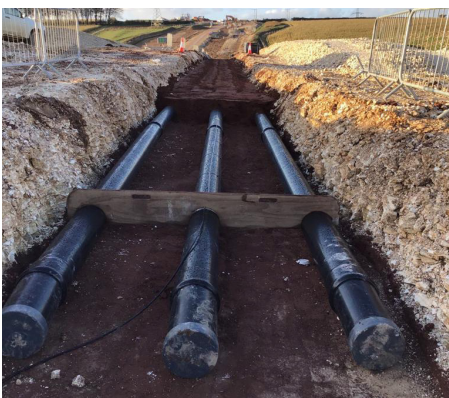
Constructing underground cable
