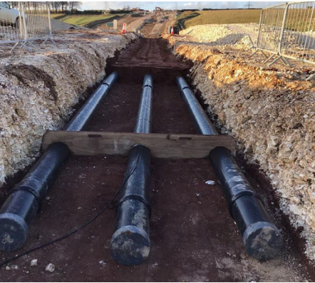
Constructing underground cable
