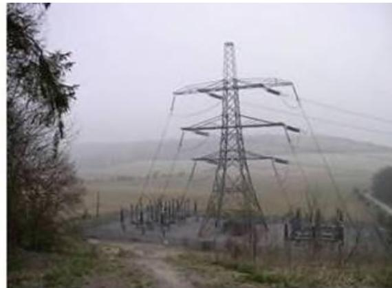
**Figure C.5: Cable Sealing End Compounds**
