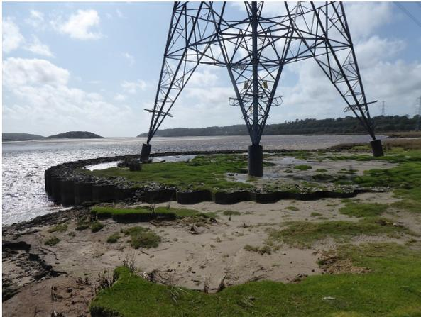
*Pylon 4ZC030R foundations and cofferdam at the edge of the estuary channel*
