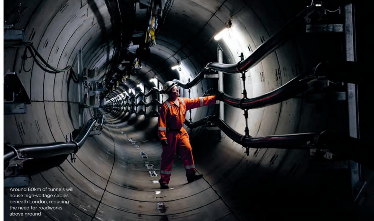
Around 60km of tunnels will house high-voltage cables beneath London, reducing the need for roadworks above ground
