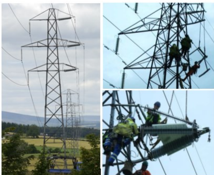
Figure 33 – Installation of RICAs on SHETL network
