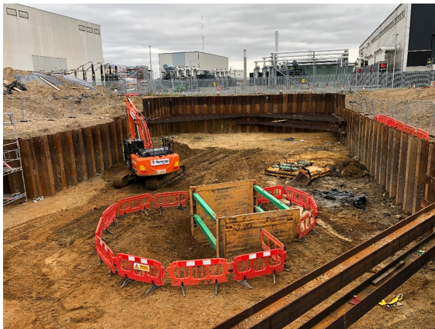
Figure 22 - Progress of Enabling Works at New Cross, October 2019
