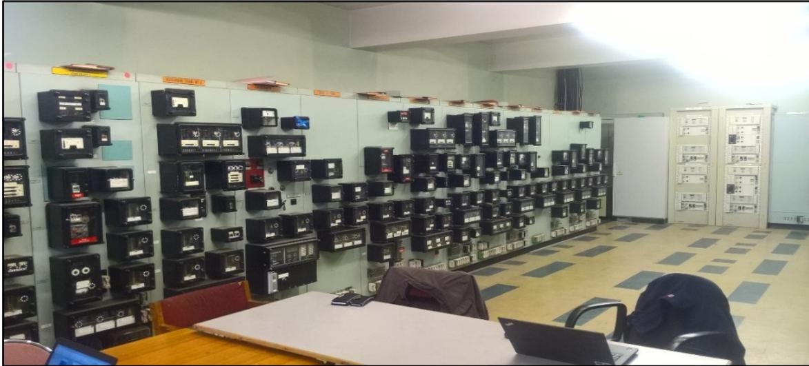
Figure 2: P&C relays at a substation
